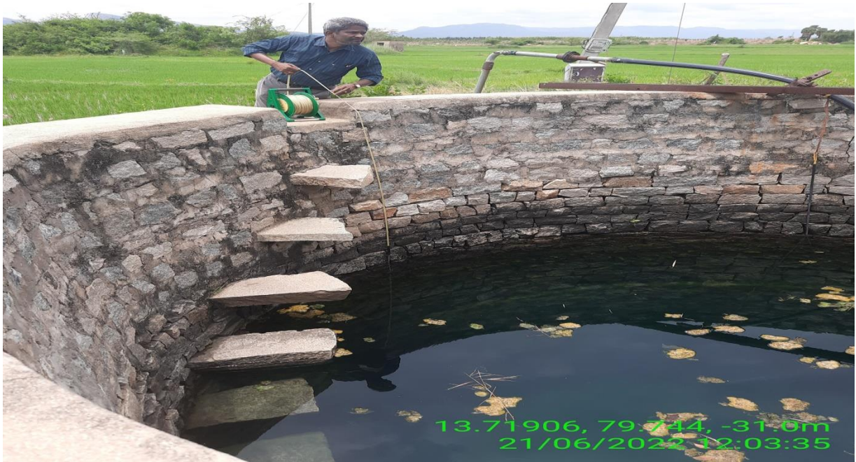
Filed Photos 4 Large Diameter dug wells used for Irrigation purposes
