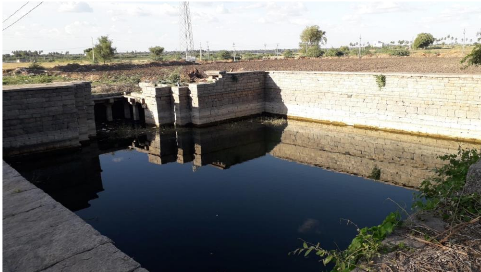
Large diameter Dug well in Satnoor village
