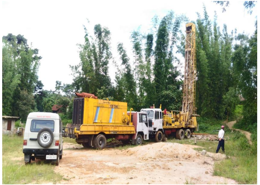
Ground Water Exploration at Mynthlu
