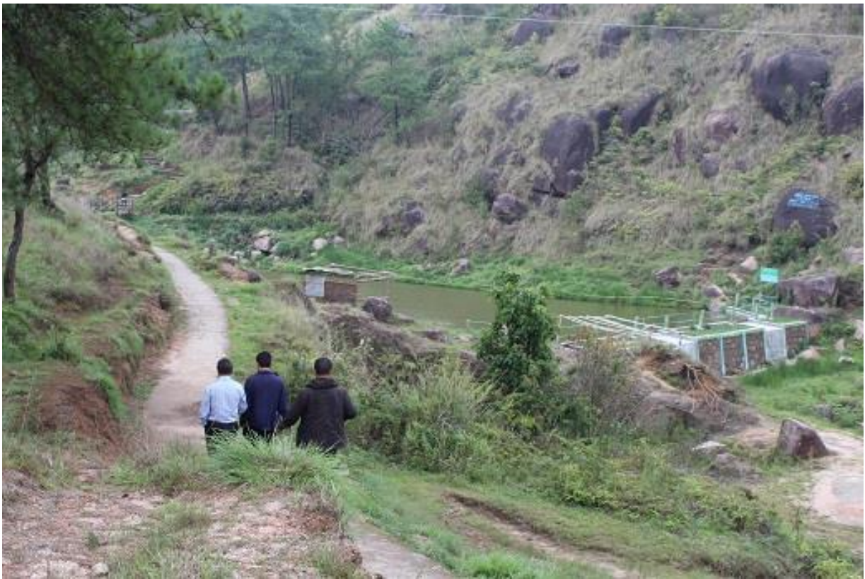
3. Water Harvesting Structure, Mawkyrwat Block
