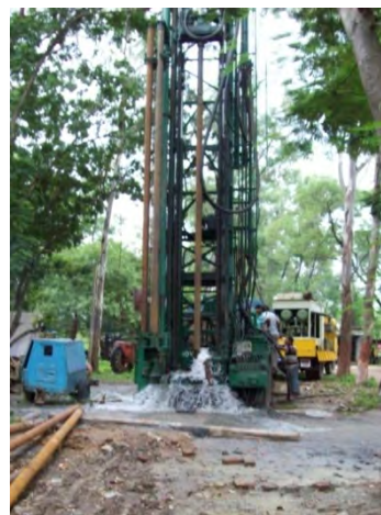
Fig 6 Rotary drilling in arsenic affected village in Bhojpur district, Bihar
