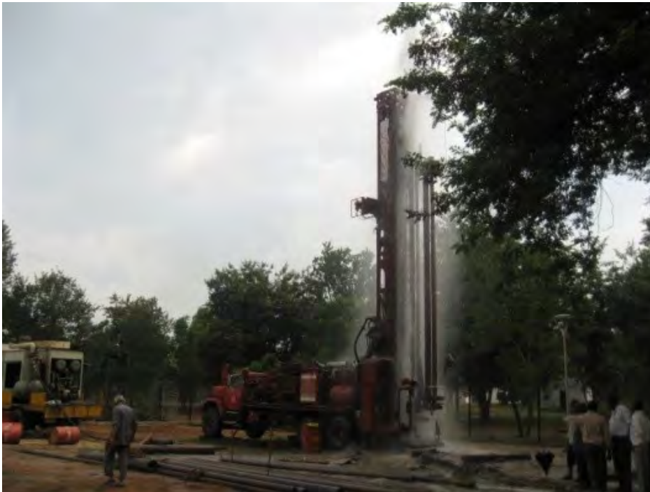
Fig 12 Drilling by DTH rig in a fluoride affected village
