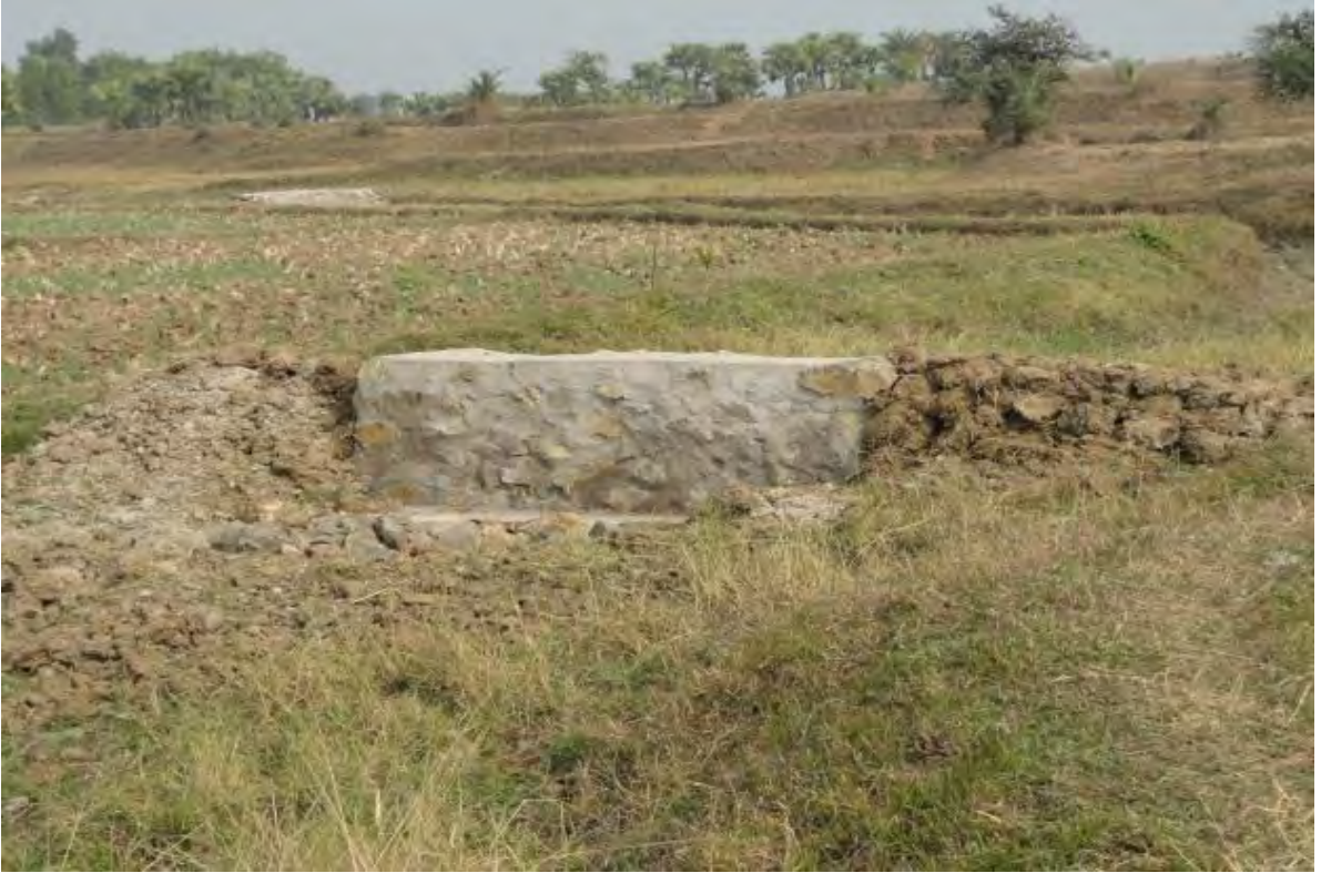
Gully Plug at Sultanpur Mouza, Nalhati-I Block, Birbhum District
