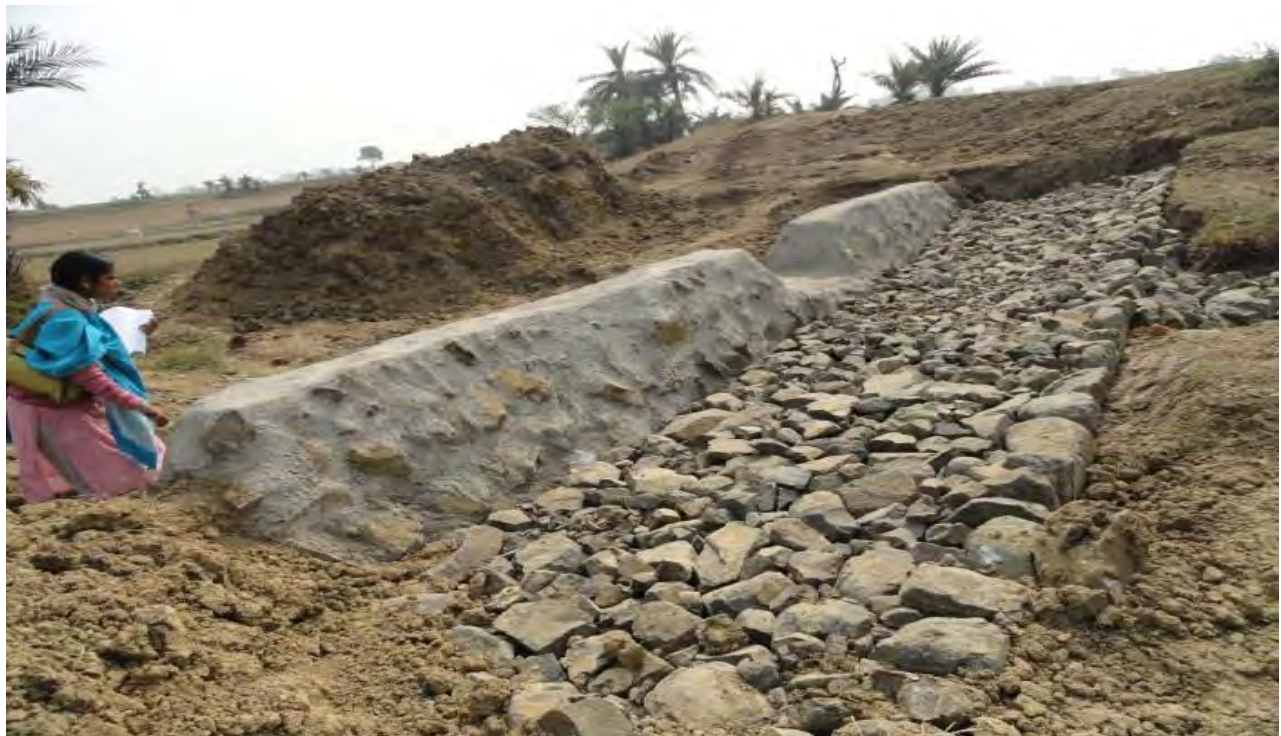
Sub-Surface Dyke at Barsor Mouza, Nalhati-I Block, Birbhum District
