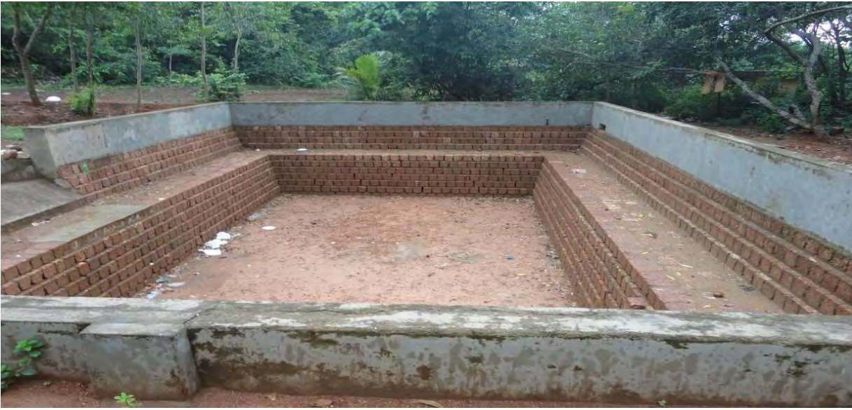
A View of Recharge Pit
