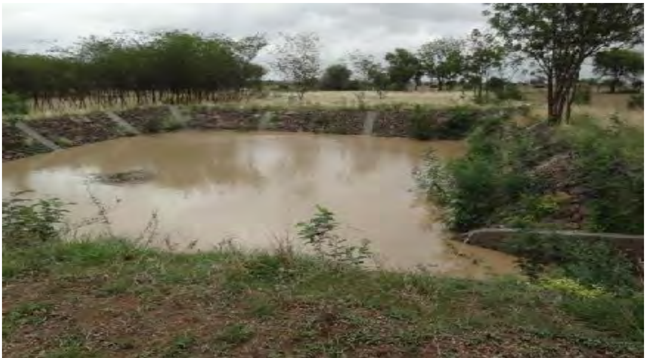
Percolation Pond after construction
