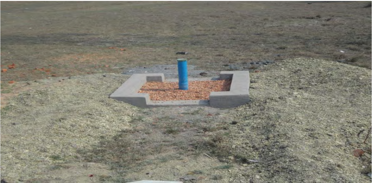
RECHARGE BORE WELLS AT BUDHAPANKA-I & II-Ligarkat Watershed, Banerpal block, AngulDist,
