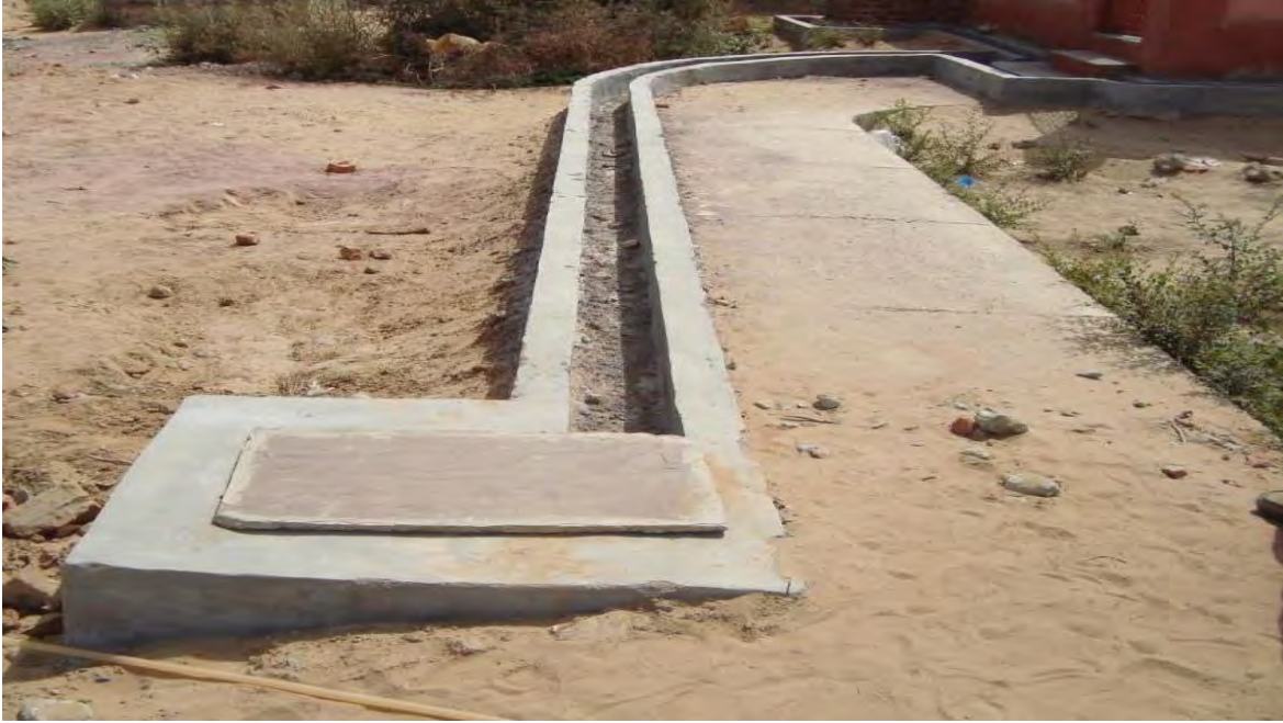
Water Channel with siphon pit. Govt. MahilaPolytechnical Collage, Bikaner city, Dist Bikaner
