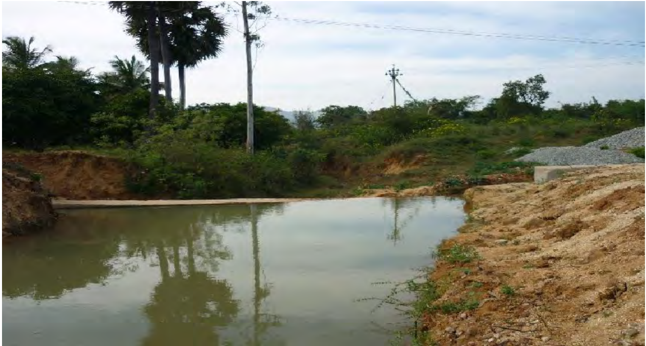
Check Dam at Karvetinagaram Village
