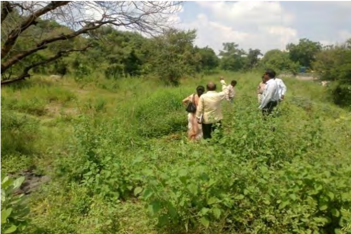
Earthen Nala Bundh -After monsoon Artificial Recharge to Groundwater in Raj Bhawan area, Nagpur, Maharashtra
