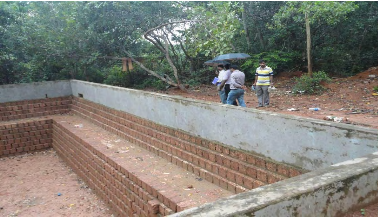
A View of Recharge Pit
