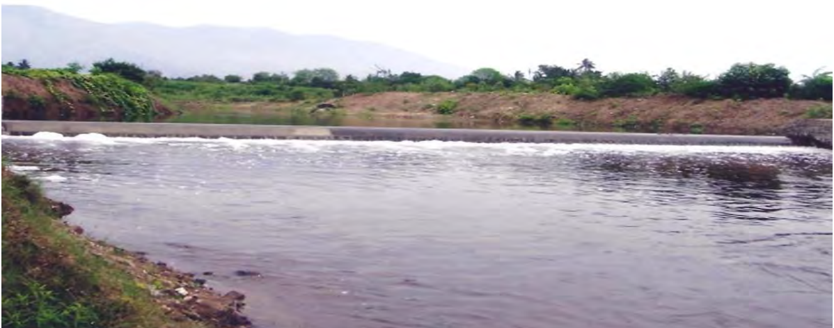
Different Stages of Construction of Artificial Recharge Structures Karuvatur watershed, NamakkalDist, Tamil Nadu
