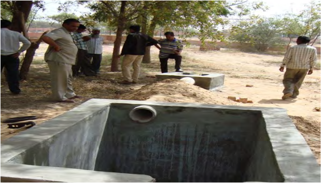
De-silting Pit- Govt. Polytechnical Collage (Boys), Bikaner city, Dist Bikaner
