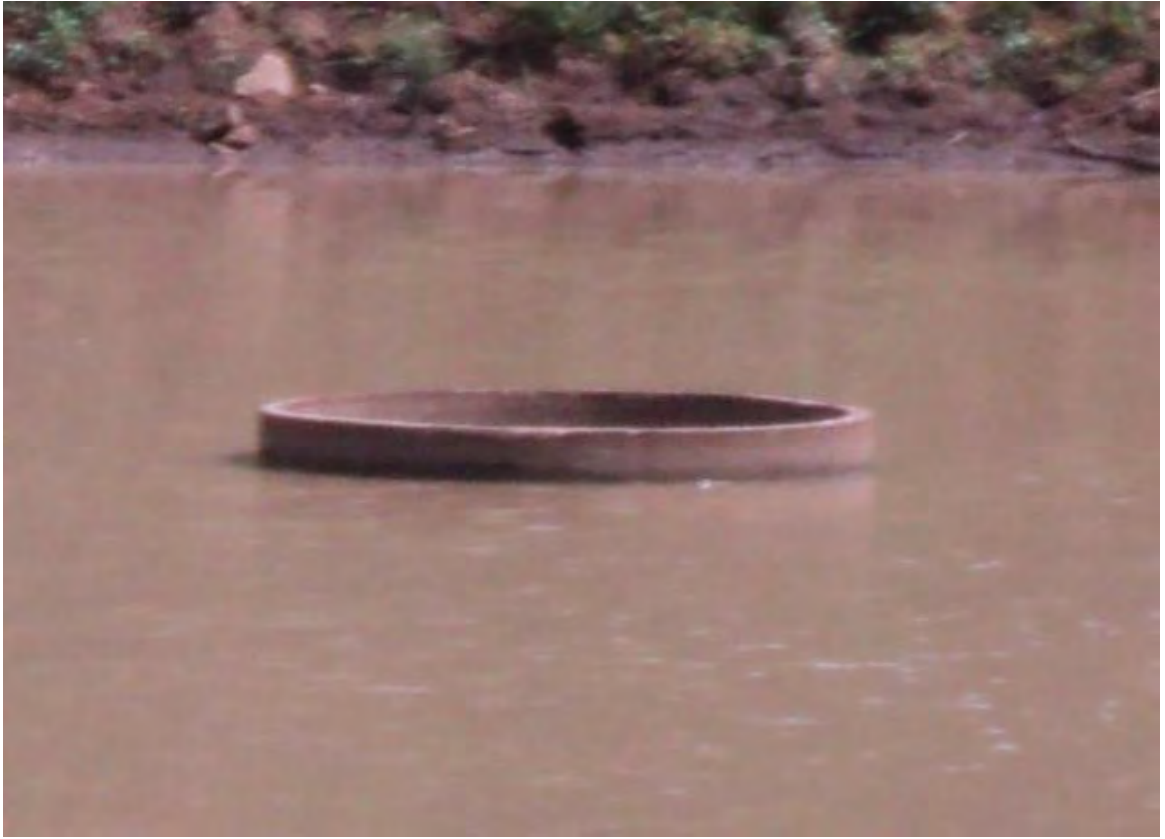
Recharge Dug Well ,Burudi Watershed, Ganjamblock,Odisha
