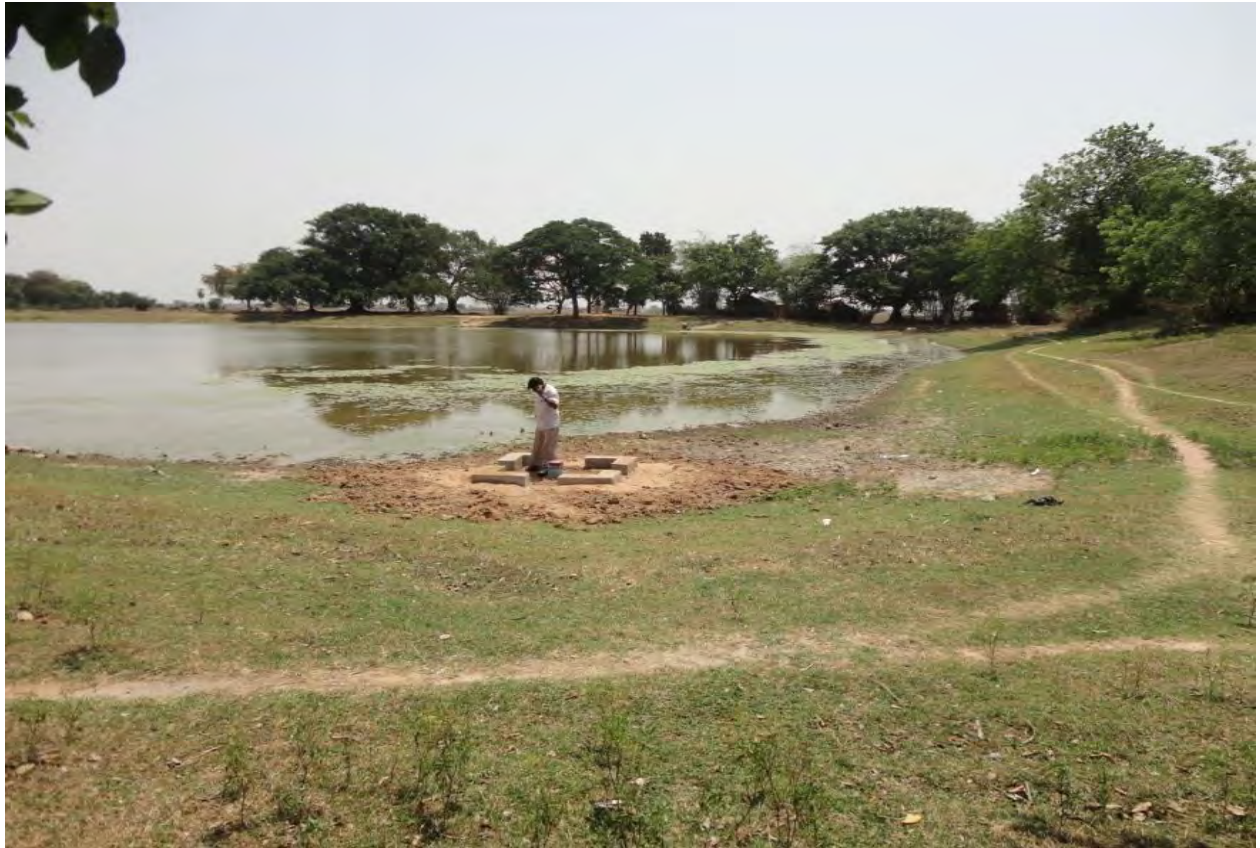
RECHARGE TUBE WELL AT BIRAMANIPUR
