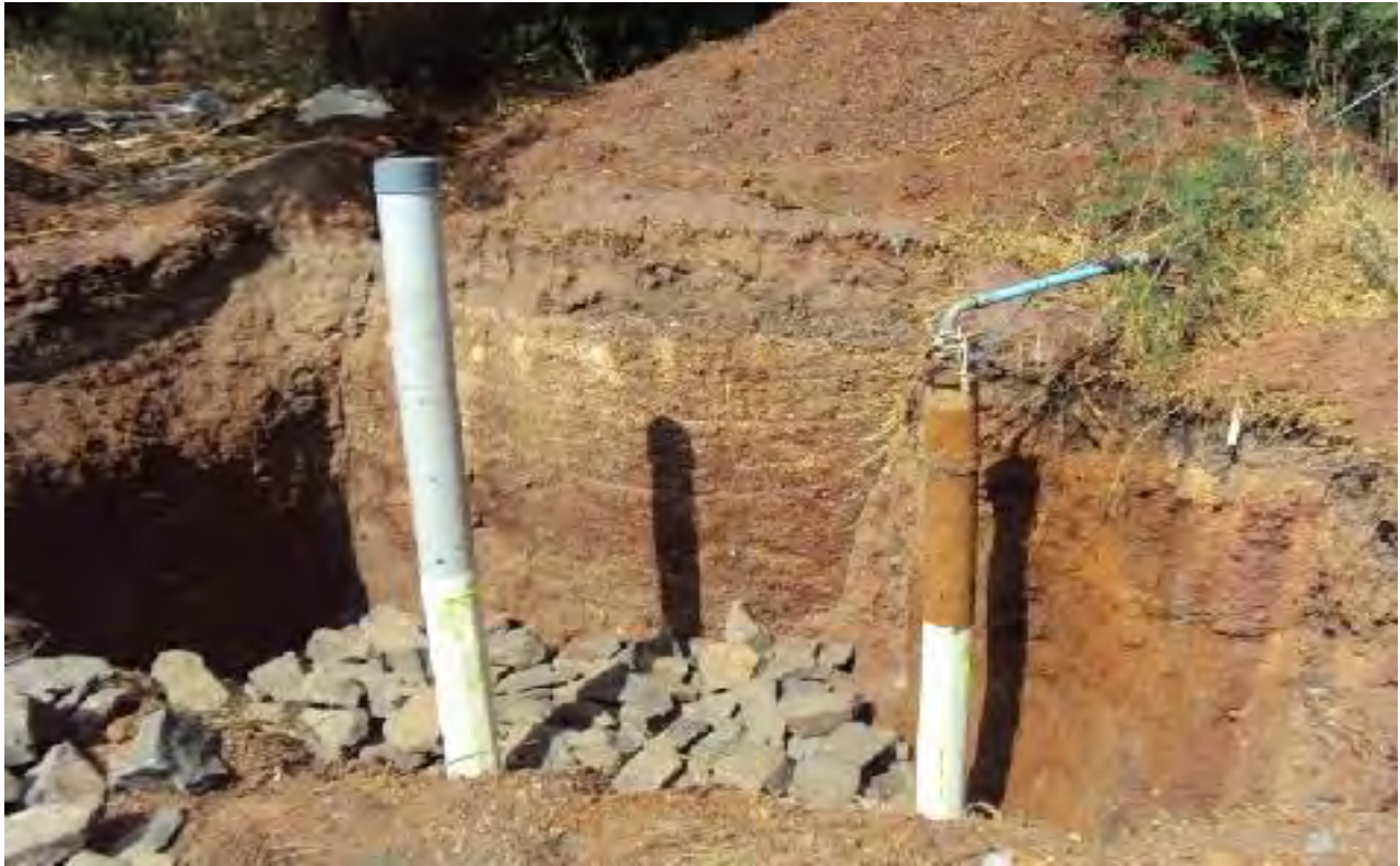
Recharge Pit Construction
