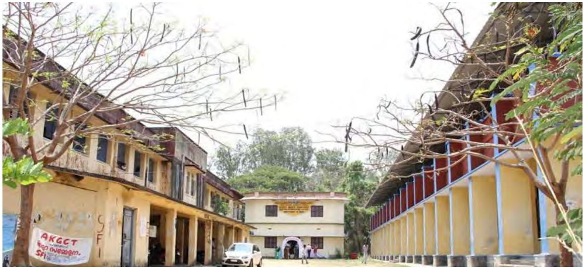
Chittur Govt. College, Palakkad Roof Top Rain Water Harvesting at Govt. college, Chittordist, Kerala
