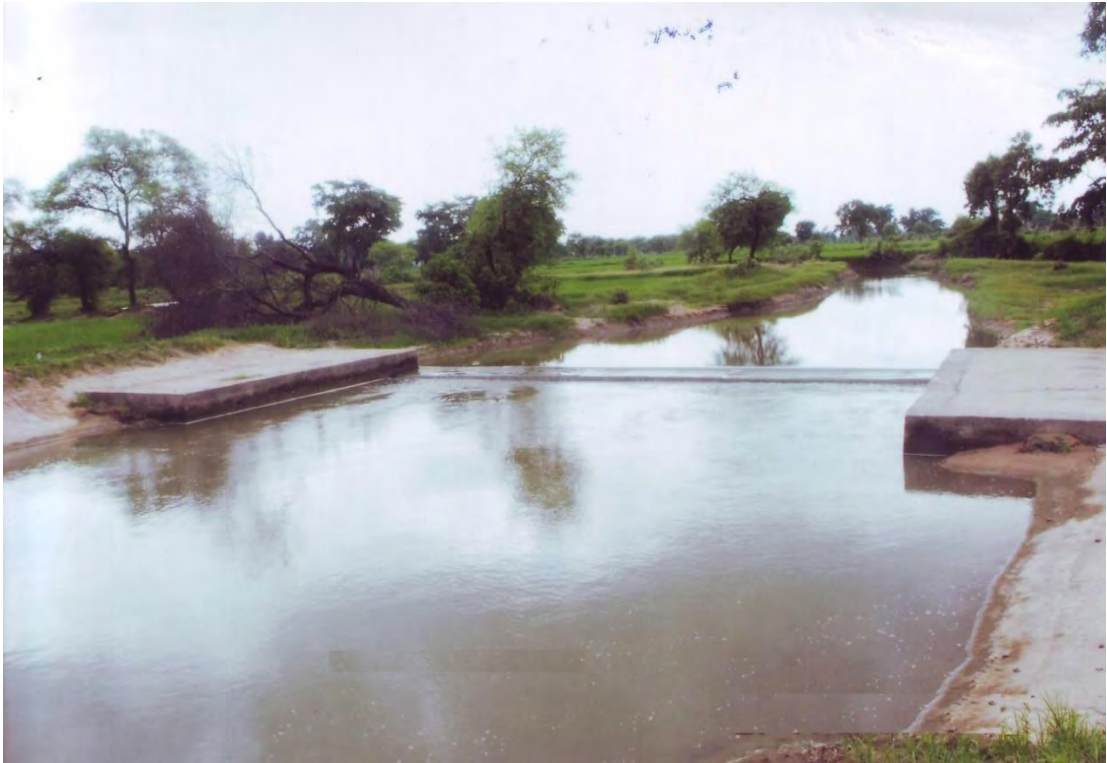
Before and after photographs of Check Dam at Devkot village no. 2 Ground Water Recharge in SanaudNala, Mili Water Shed, Block Gurur district Durg
