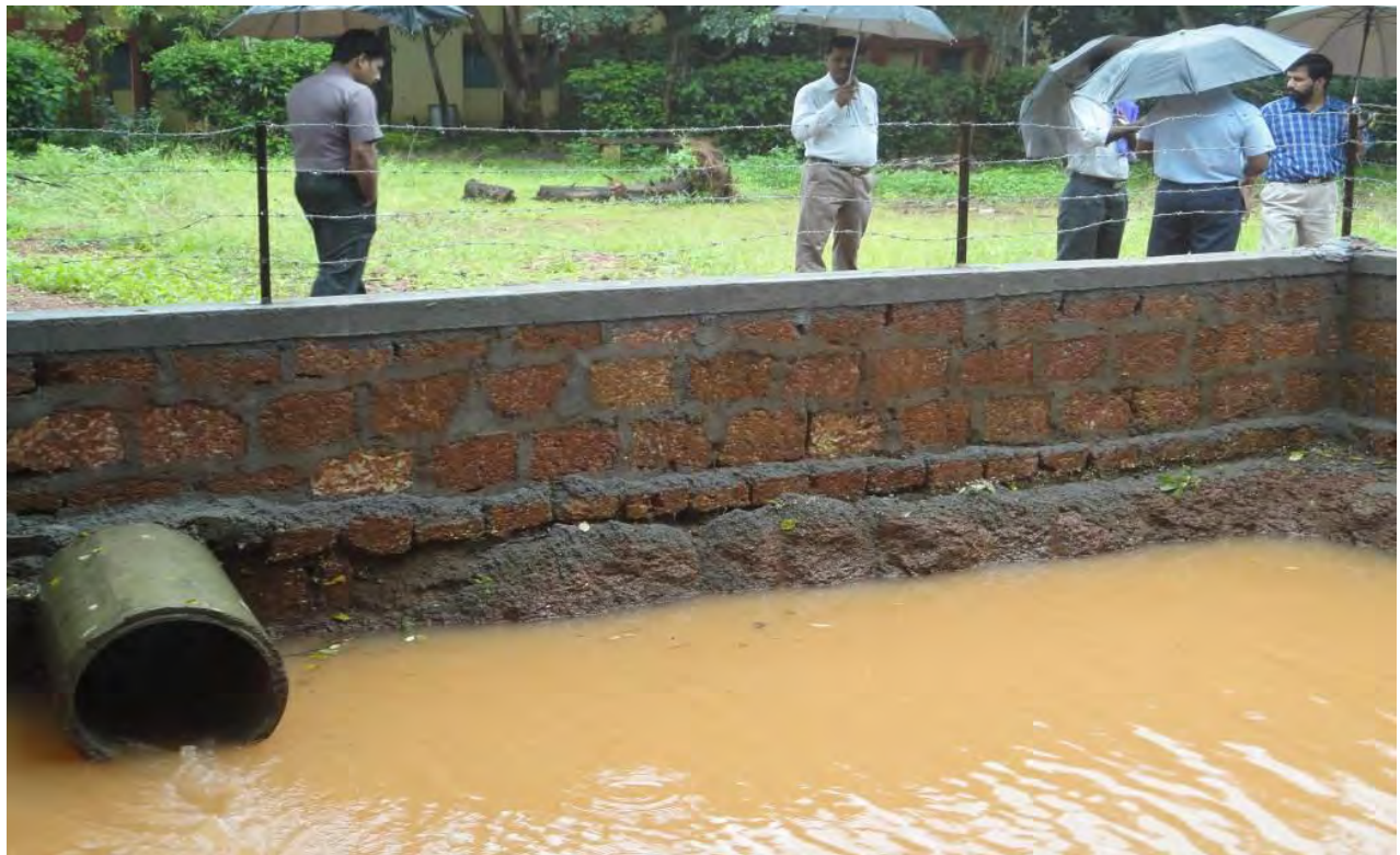
A view of flowing water through drainage channel to Recharge Pit
