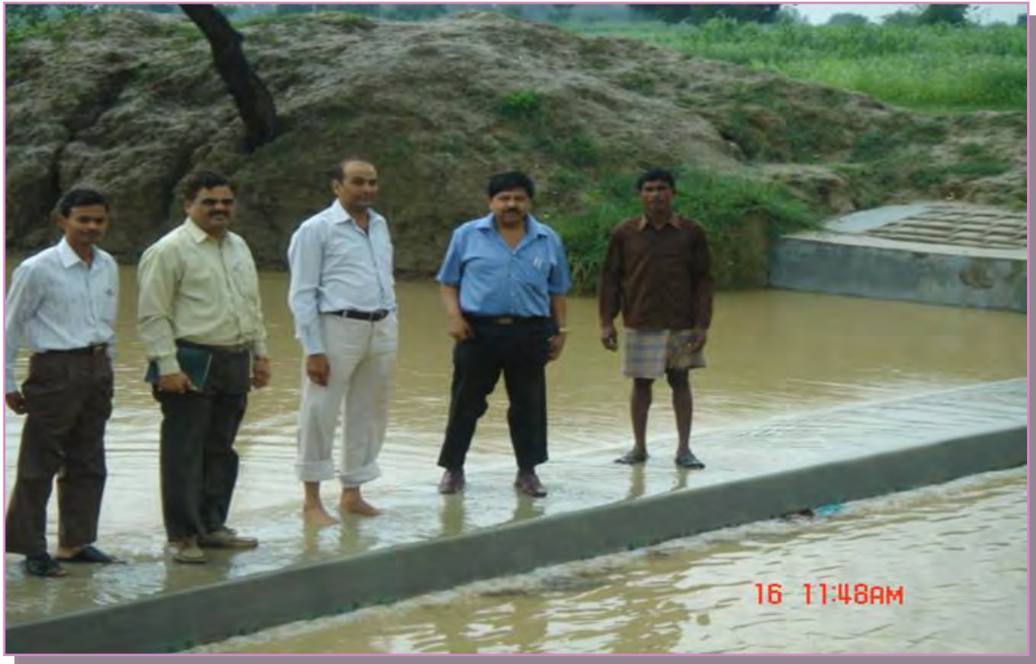
CHECK DAM AT SATAON BLOCK, DISTRICT RAEBARELI, UP
