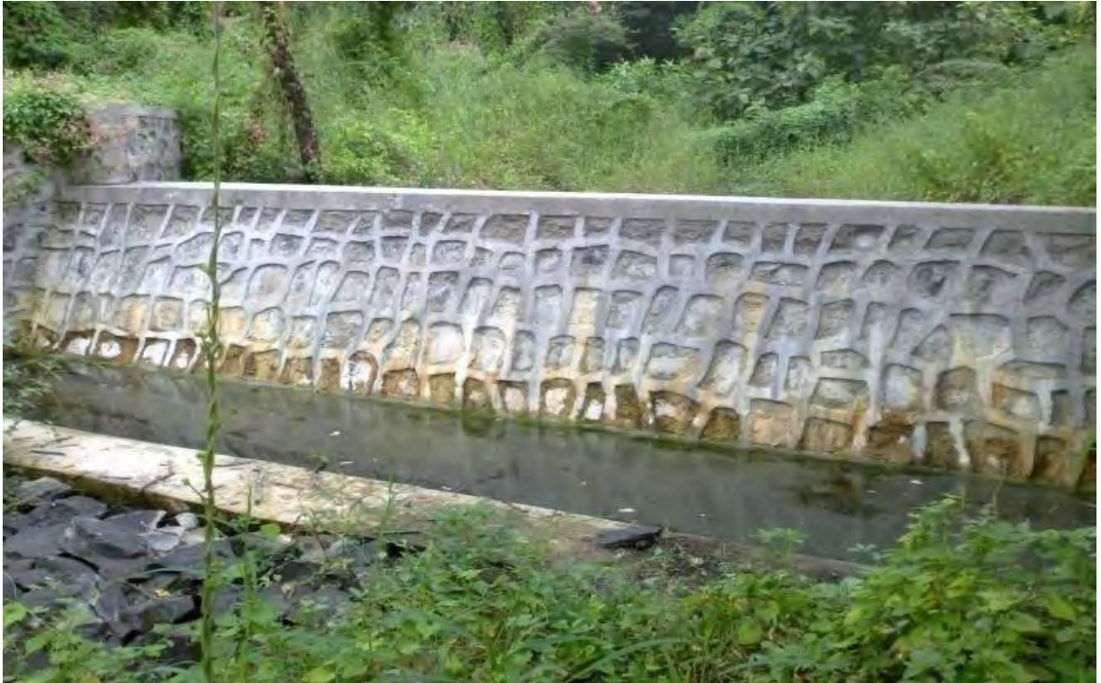
Cement Nala Bundh -After monsoon Artificial Recharge to Groundwater in Raj Bhawan area, Nagpur, Maharashtra
