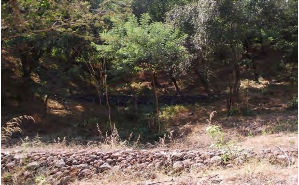
Gabion Structure-Before monsoon
