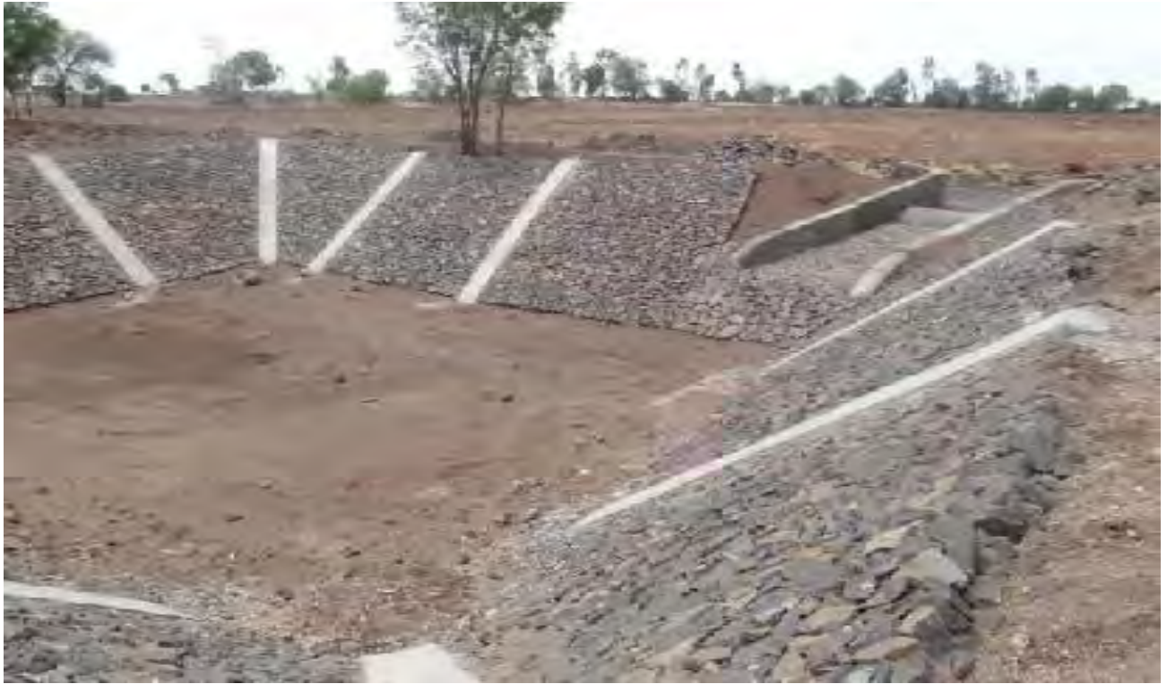
Percolation Pond under construction
