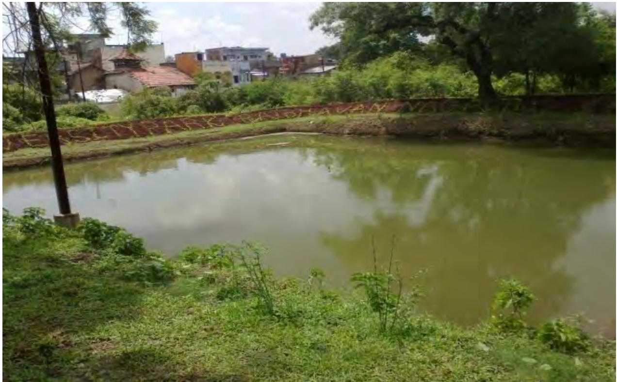
Filled up Farm ponds-Repetitive filling of pond during the monsoon Artificial Recharge to Groundwater in Raj Bhawan area, Nagpur, Maharashtra
