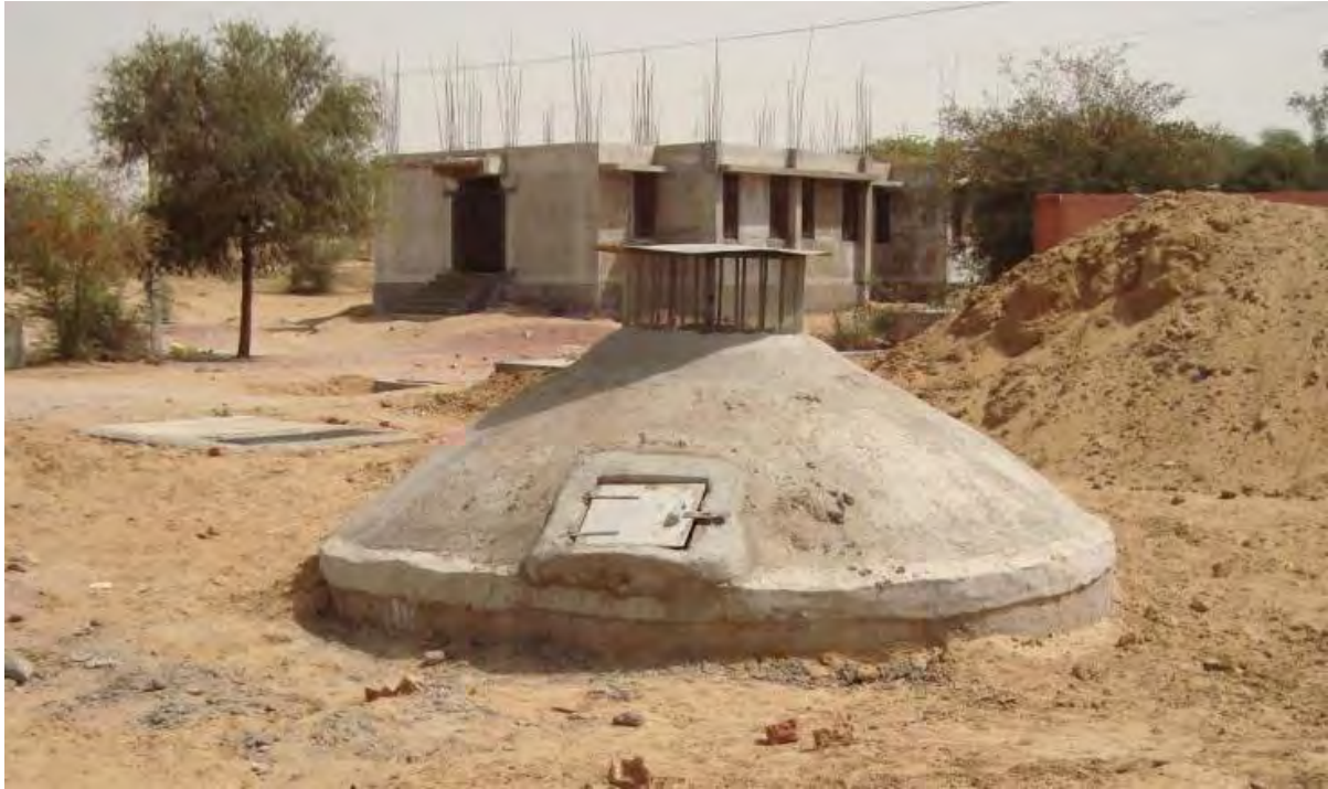
Reservoir (collection) Tank Govt. MahilaPolytechnical Collage, Bikaner city, Dist Bikaner
