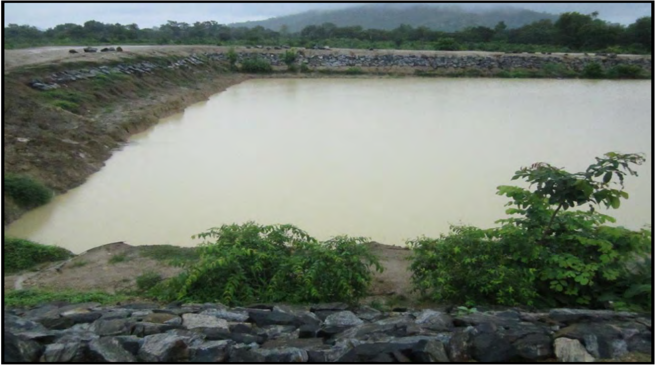
PERCOLATION TANK- Karmeli mini Watershed ,Saintala block, Bolangirdist, Odisha
