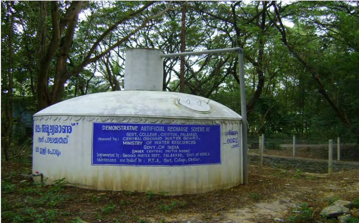
A view of the functional Ferro Cement Tank with Recharge Pit
