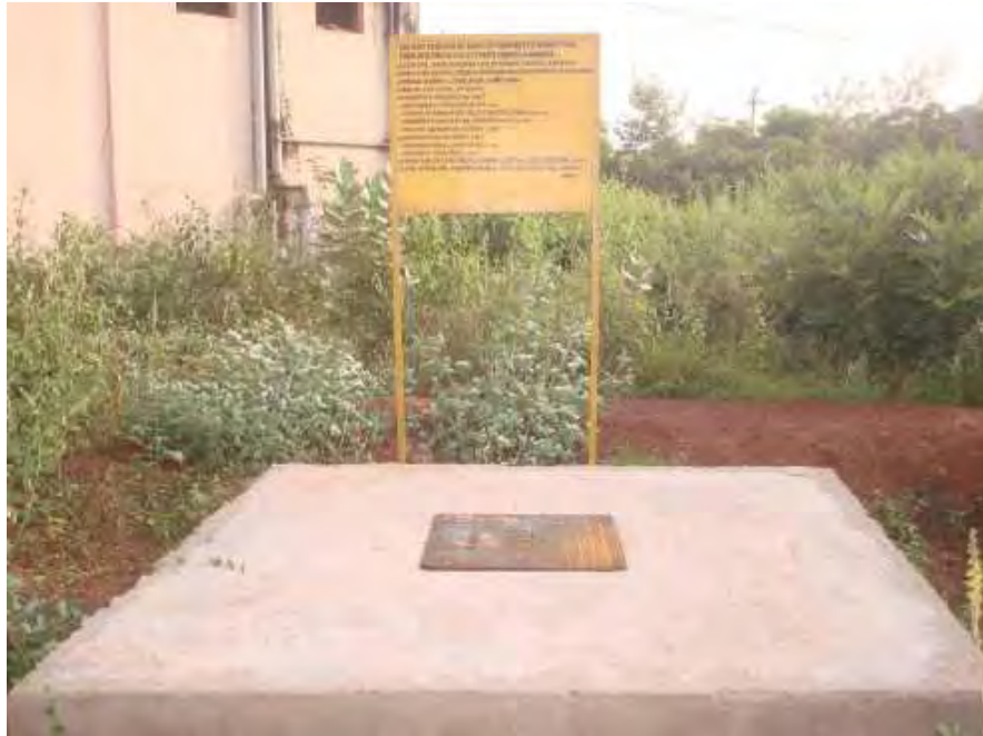
[RECHARGE BORE WELL INSTALLED IN DRDA OFFICE CAMPUS] OFFICE BUILDING, COLLECTORATE CAMPUS, KHURDA DIST
