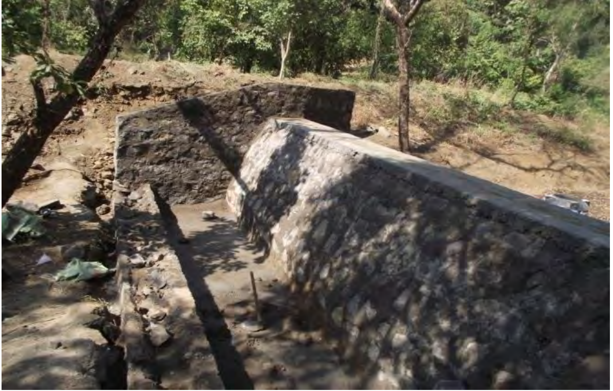
Cement Nala Bundh-Before monsoon
