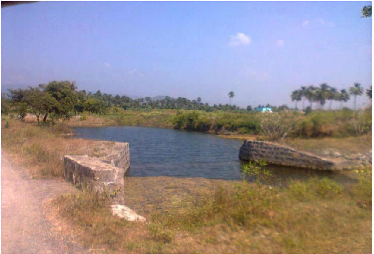
Kattukottai Percolation Pond-Thalaivasal Block, Selam District, Tamil Nadu
