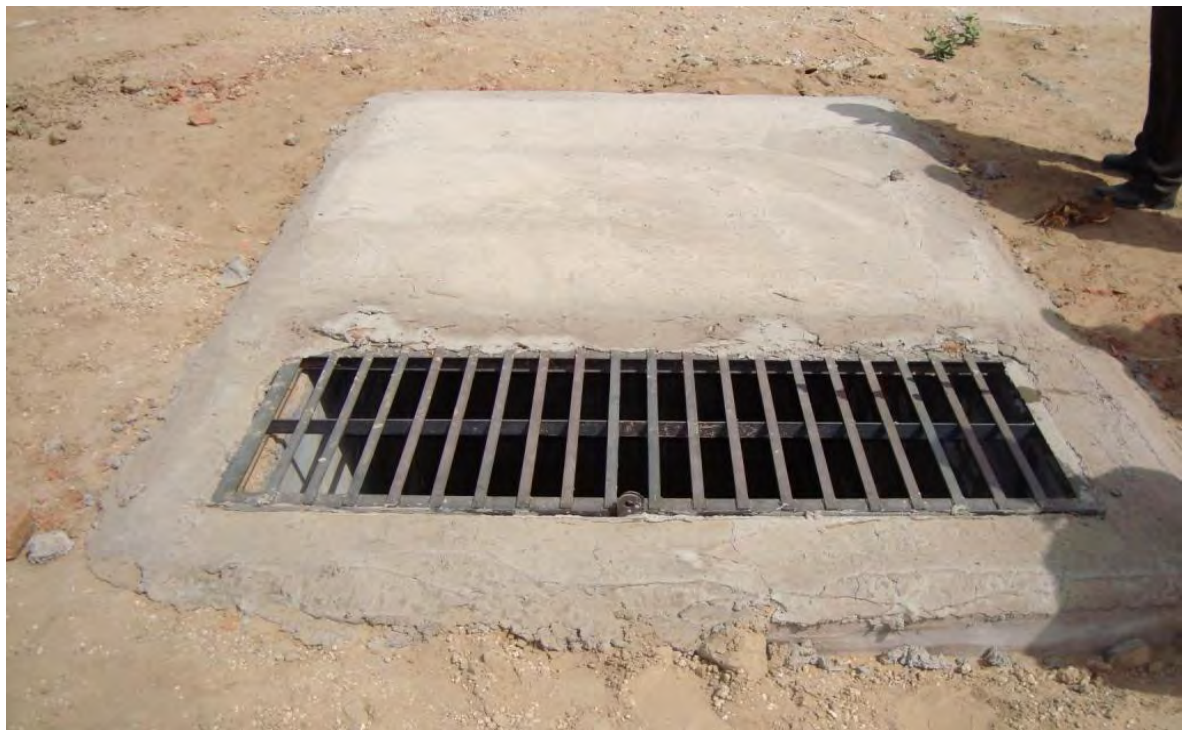
De-silting Pit Govt. MahilaPolytechnical Collage, Bikaner city, Dist Bikaner
