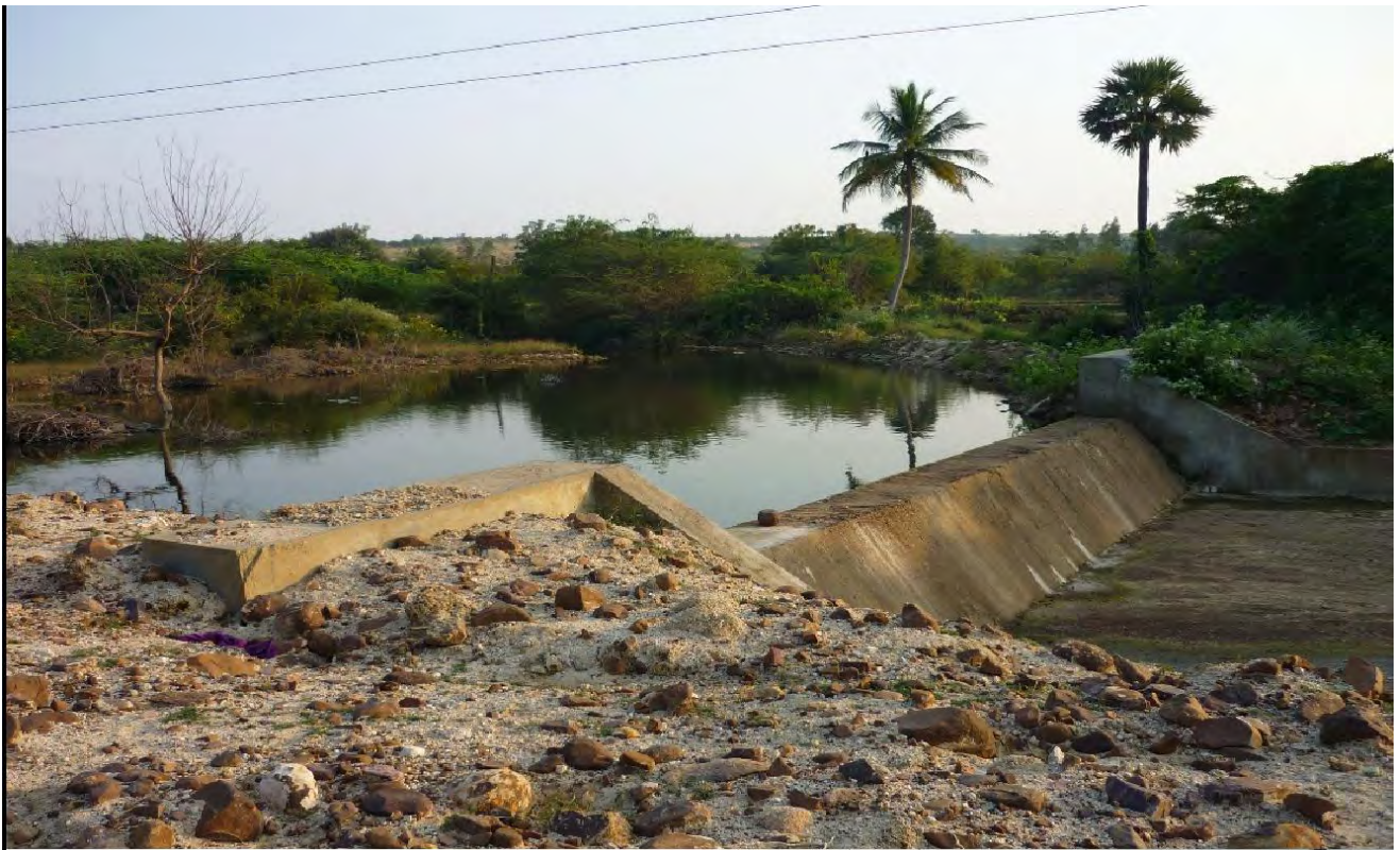
Check Dam at Mittoor Village Artificial Recharge Structures on ground water in Chittoor District, Andhra Pradesh
