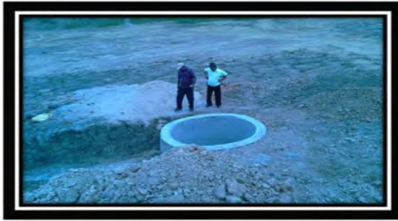
Recharge well in Existing pond Village : Vyasvasna Ta- Kapadvanj Under Construction
