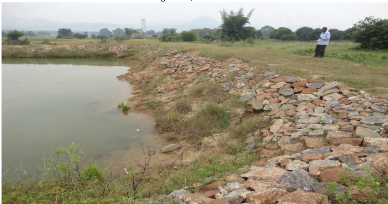
RECHARGE TANK AT ANGAPADA Himtira Watershed, Kishornagar block AngulDist, Odisha
