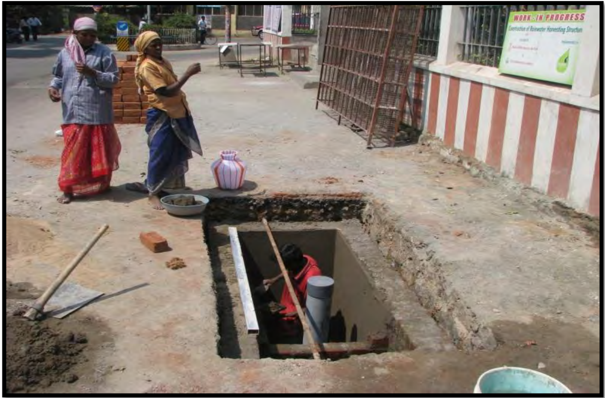
Rectangular Structure- RWHS in Coimbatore city, Coimbatore Block, Dist. Coimbatore, Tamil Nadu
