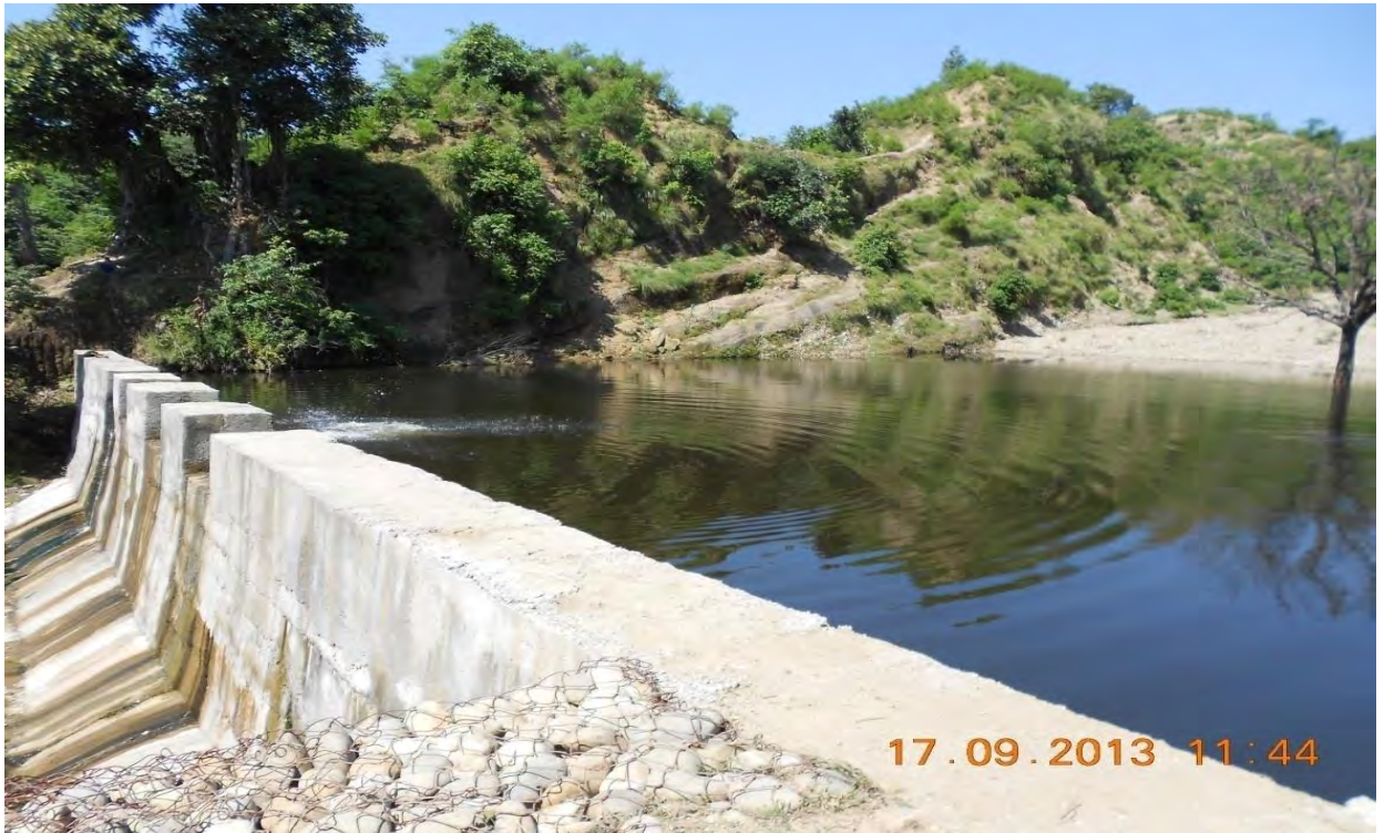
CHECK DAM AT PHANGERI, KATHUA
