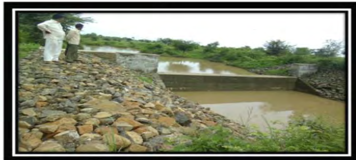
Renovation of Check Dam (After) Village : Viraniya Ta- Kapadvanj
