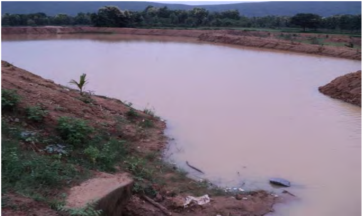
Post-Project Recharge Tank, Burudi Watershed, Ganjamblock, Odisha
