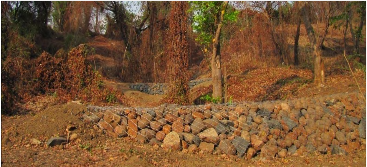
Gabion Structure-Before monsoon
