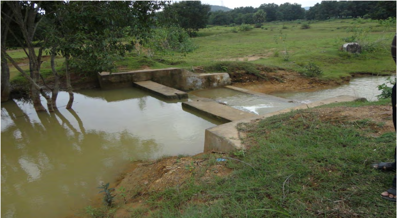
CHECK DAM AT TURUDA-Himtira Watershed, Kishornagar block AngulDist, Odisha
