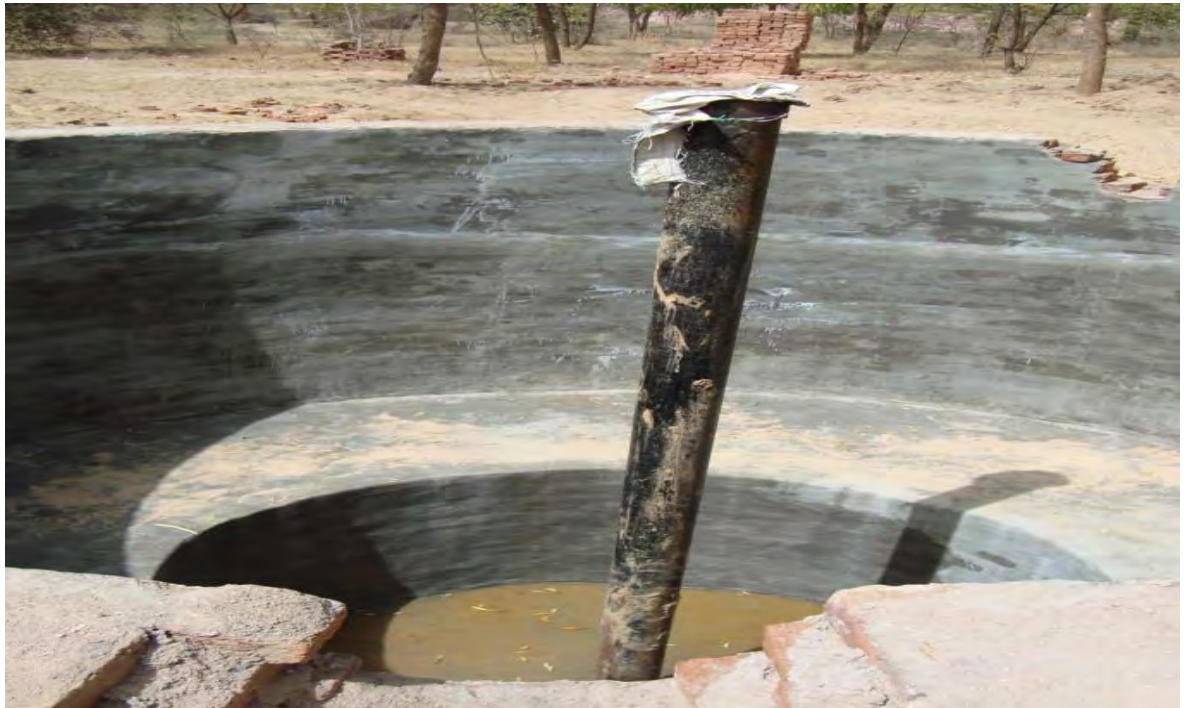
Circular Recharge Pit with filter pit & recharge tube well Govt. Polytechnical Collage (Boys), Bikaner city, Dist Bikaner
