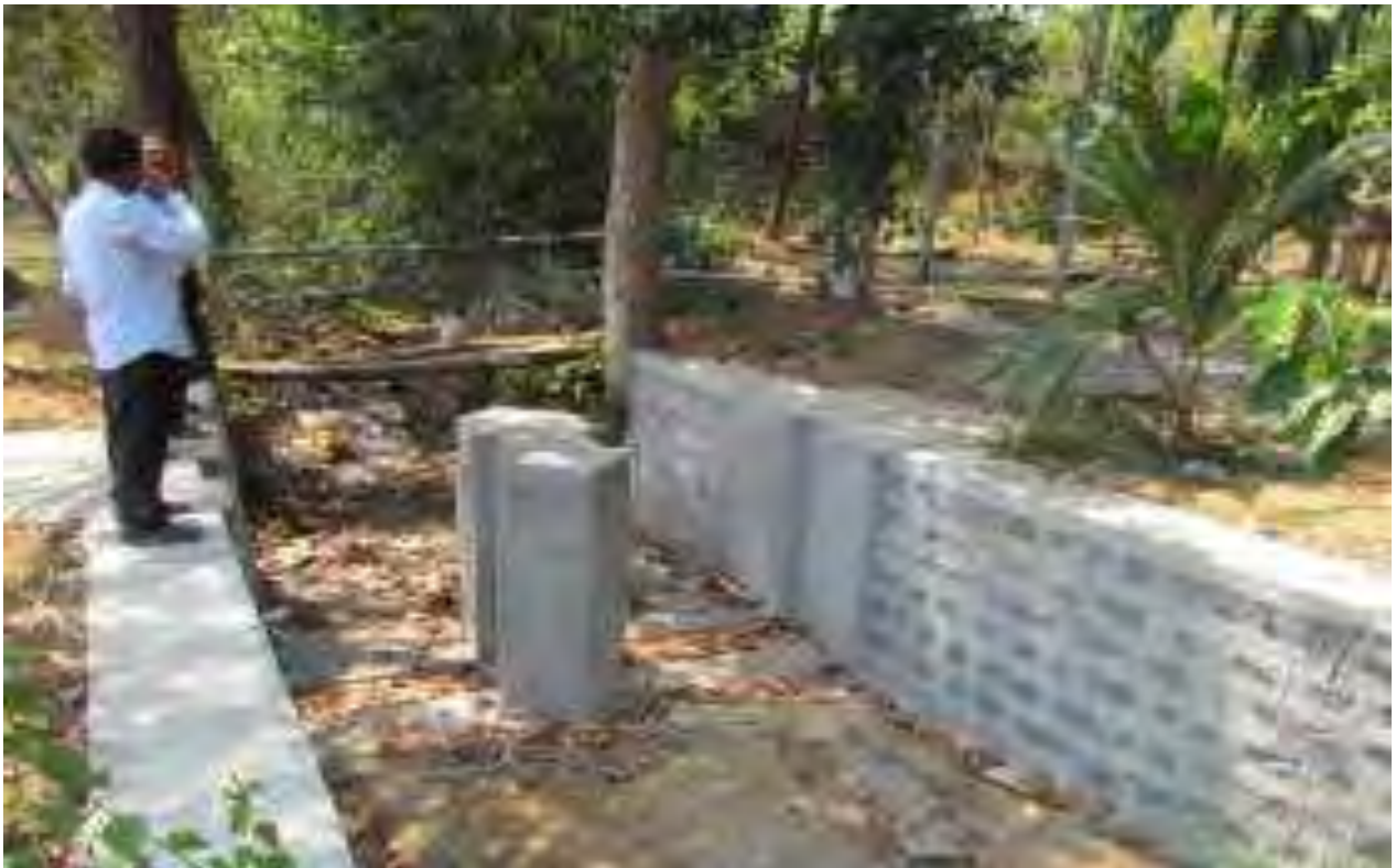
Vented Dams constructed in Panemangalore Sub-watershed
