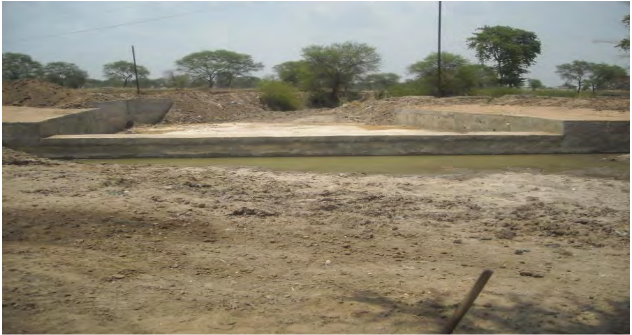
Check Dam at village Kanwar
