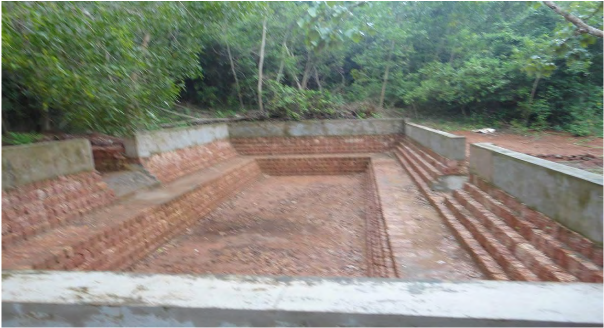
A View of Silt Collection Tank
