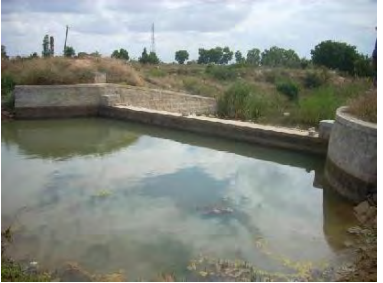
Percolation Tank constructed at Malur Taluk
