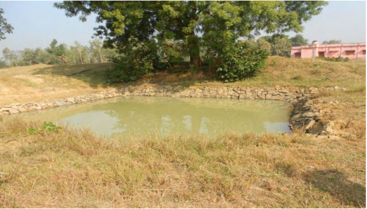
RECHARGE TANK -Karmeli mini Watershed ,Saintala block, Bolangirdist, Odisha
