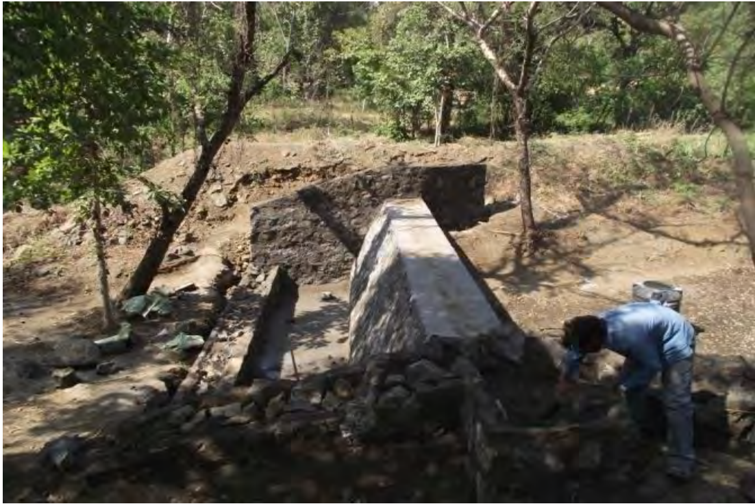
Cement Nala Bandh-Before monsoon
