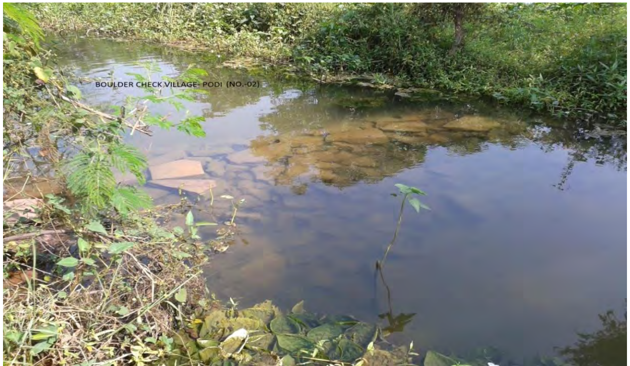
Boulder Check dam at Podi
