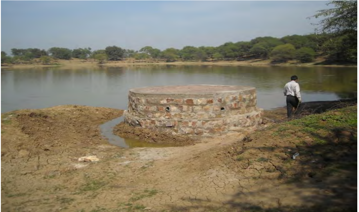
Recharge Shaft no. 1 at village Kanwar
