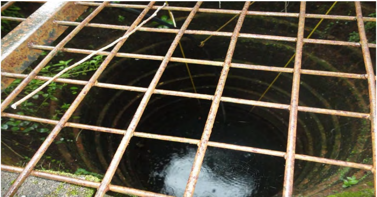
A View of School supply well
