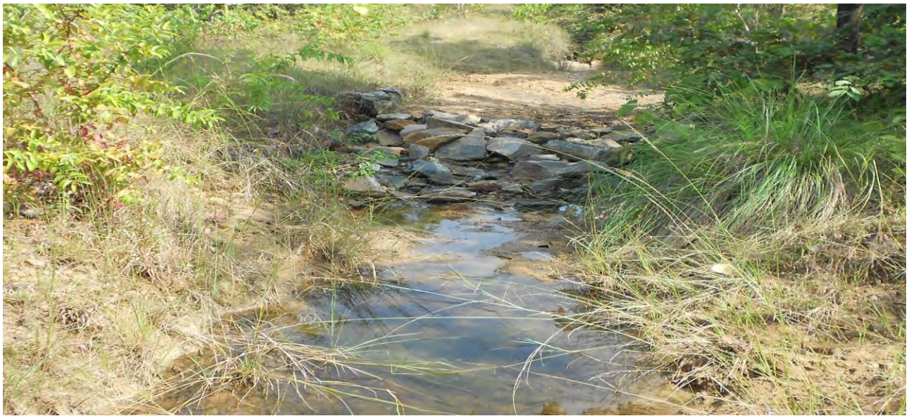
LOOSE BOULDER CHECK DAM--Karmeli mini Watershed ,Saintala block, Bolangirdist, Odisha
