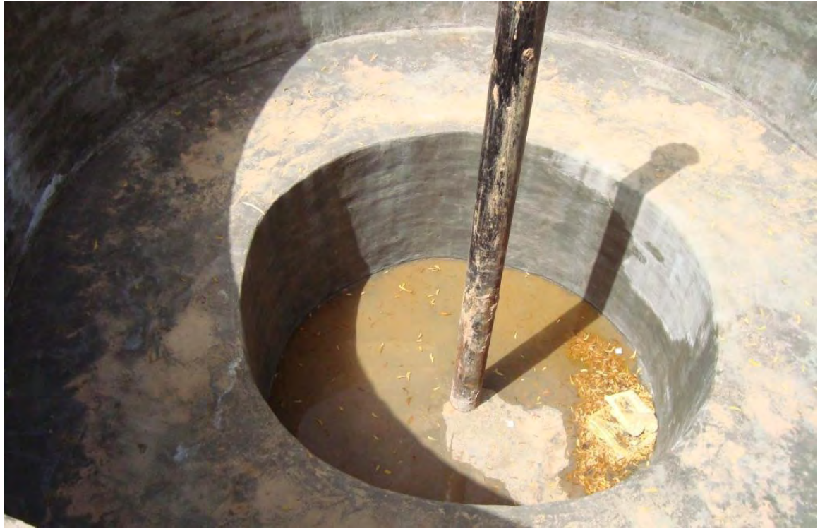
Circular Recharge Pit with filter pit & recharge tube well Govt. Polytechnical Collage (Boys), Bikaner city, Dist Bikaner
