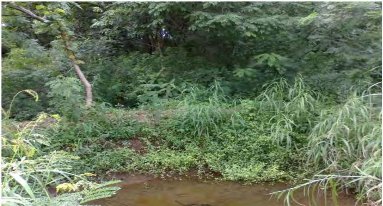
Gabion Structure-After monsoon
