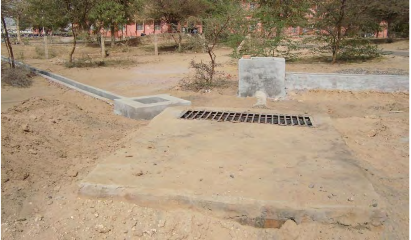
De-silting Pit-CE, IGNP Office Building, Bikaner city, Dist Bikaner
