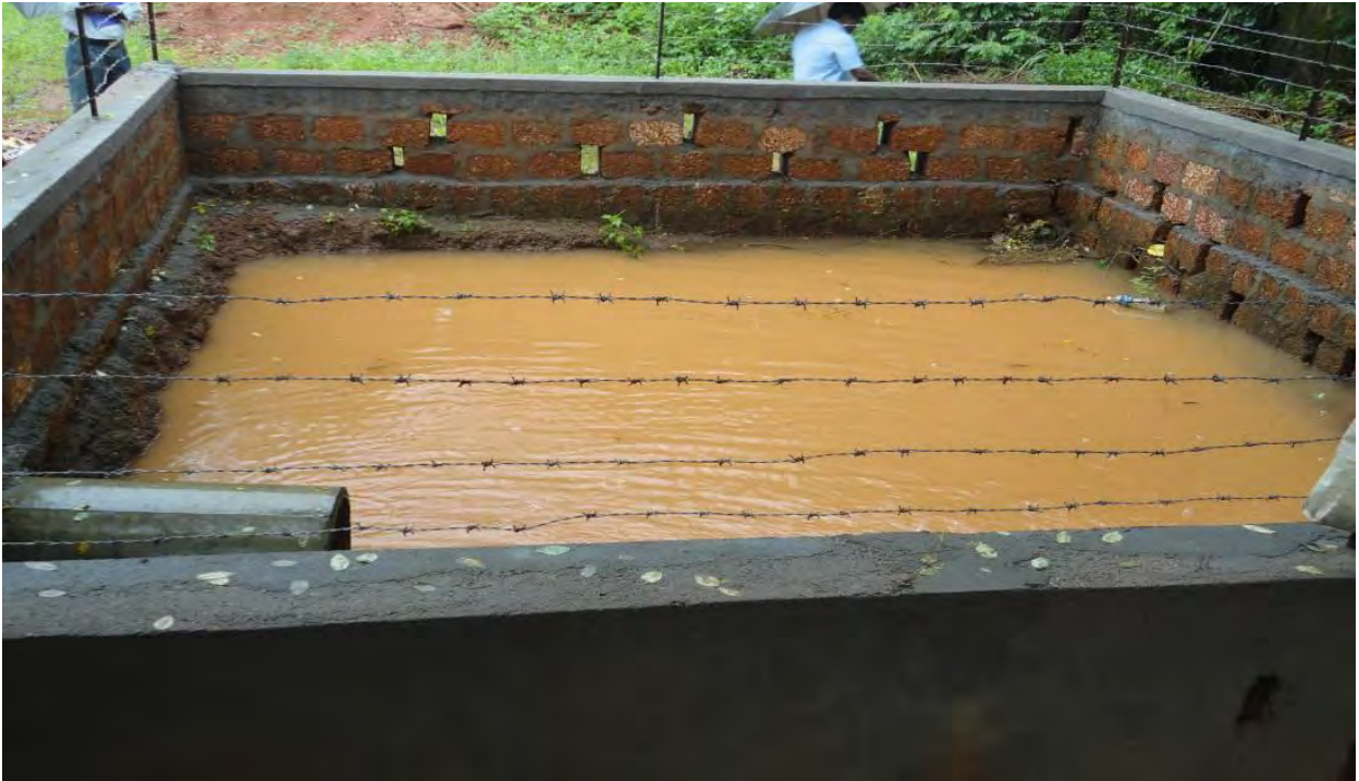
A View of Recharge Pit with collected Rain Water
