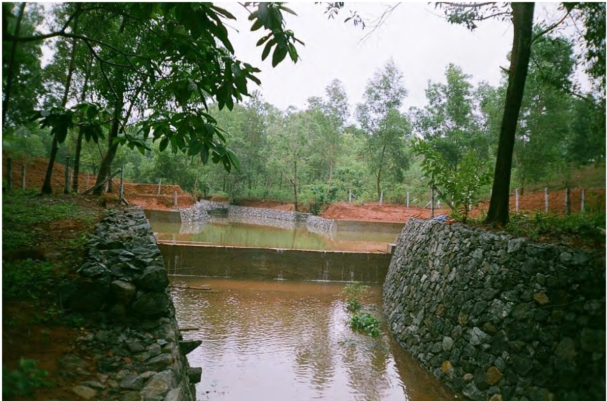
Check Dam, Artificial Recharge in ManjeshwarGovindPai Memorial College campus Kasargod, Kerala
