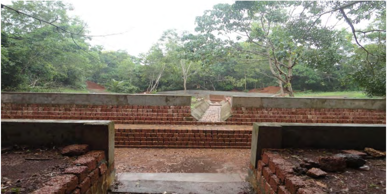
View of Drop pit
