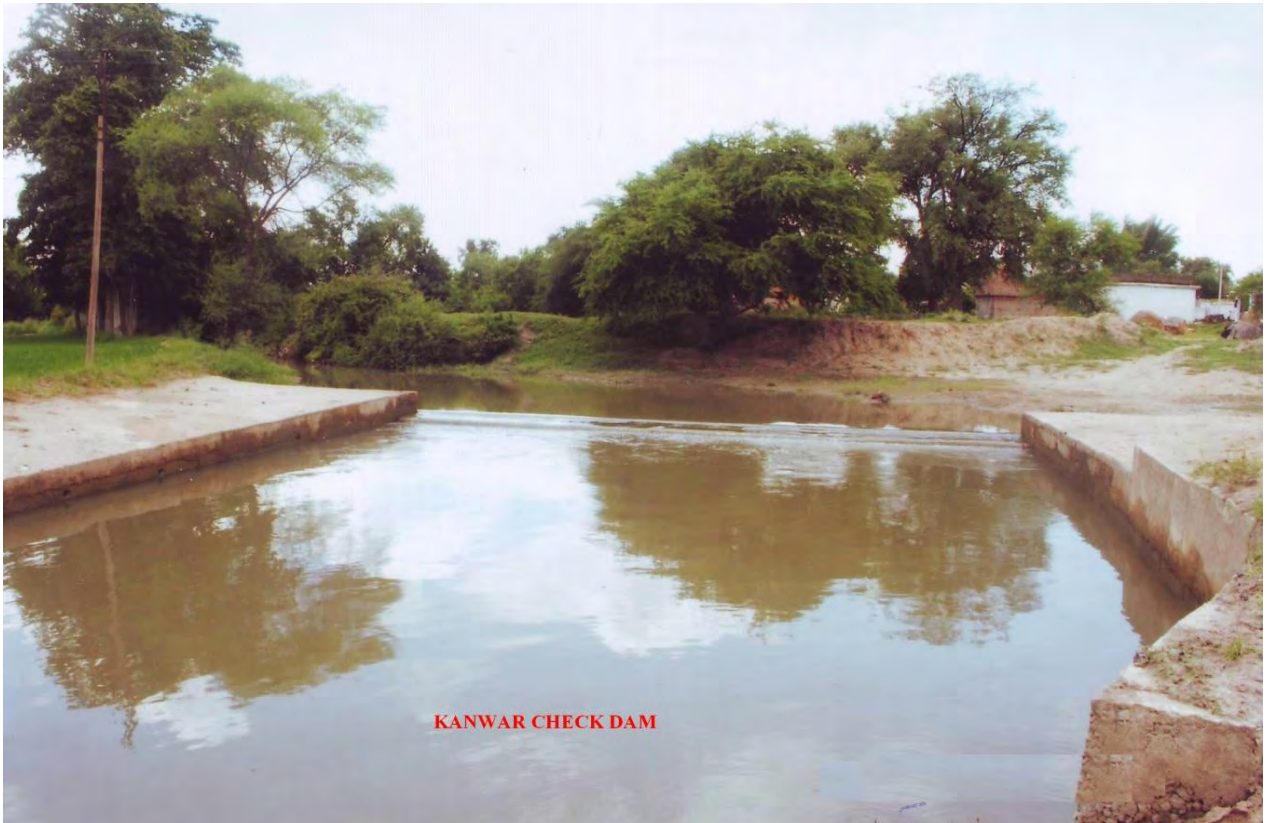
Surface run off arrested at Check Dam, Kanwar Ground Water Recharge in SanaudNala, Mili Water Shed, Block Gurur district Durg
