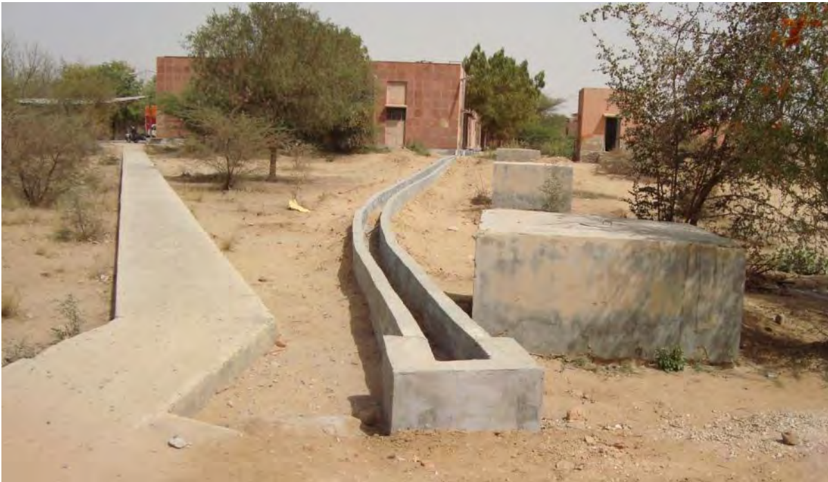
Water Channel with siphon pit. Govt. MahilaPolytechnical Collage, Bikaner city, Dist Bikaner
