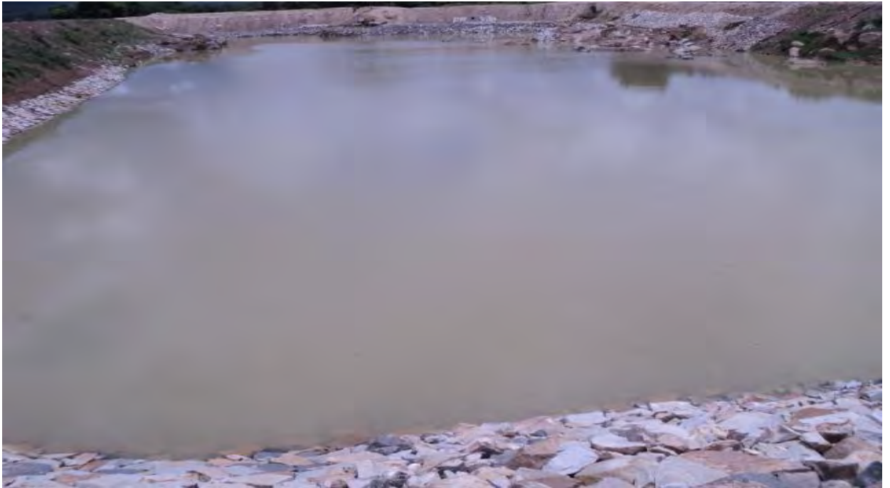
Post-Project Recharge Tank, Burudi Watershed, Ganjamblock, Odisha
