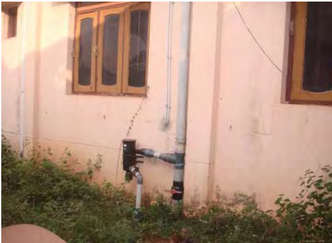
[ON-LINE FILTER INSTALLED] OFFICE BUILDING, COLLECTORATE CAMPUS, KHURDA DIST
