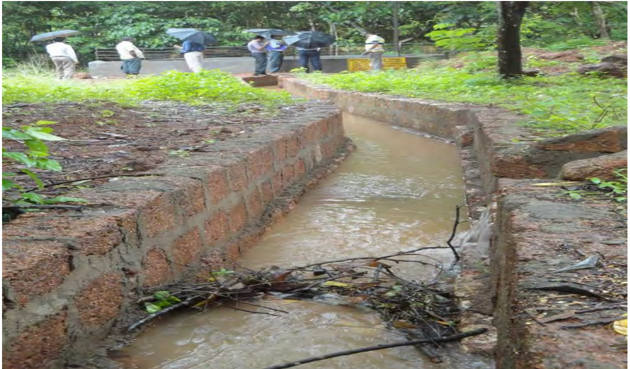
A view of flowing water through drainage channel to Recharge Pit
