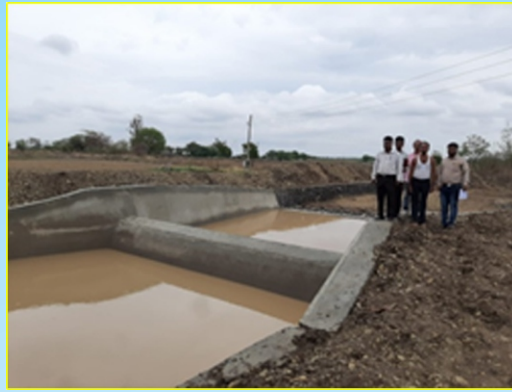
Water filled up in first rain in check dam in Osmanabad.
