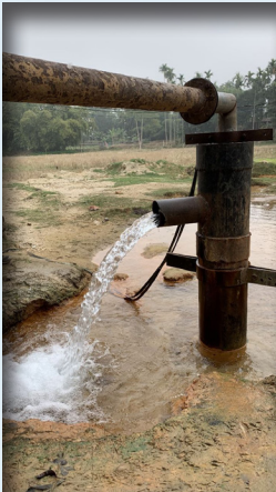
Auto flow well (discharge of 14.6lps) at Char Ganki
