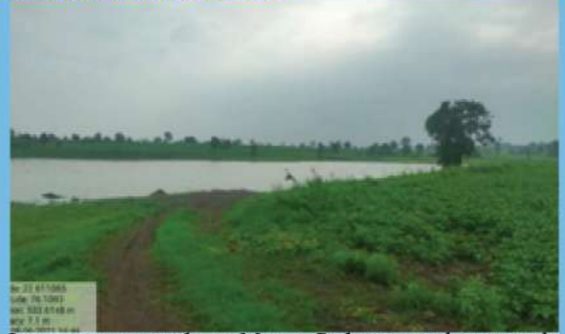
Interventions made in Mogya Pedme percolation tank, Indore, Madhya Pradesh
