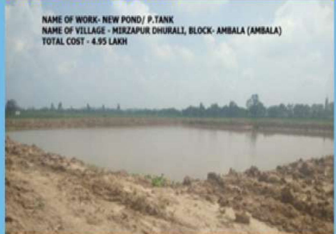
Interventions made in Check dams and ponds in Ambala district.
