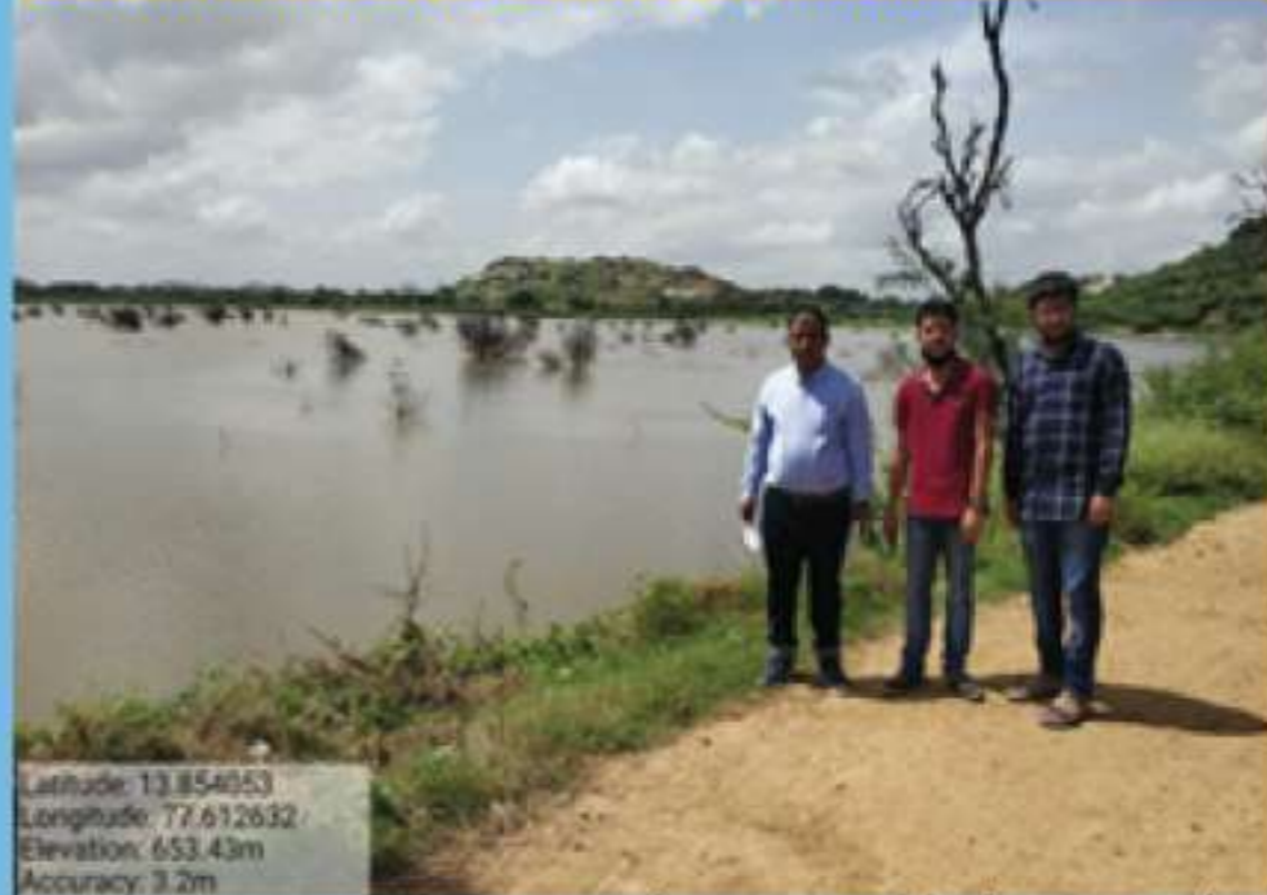
Interventions made in Kondur water Tank at Kondur, Lepakshi mandal
