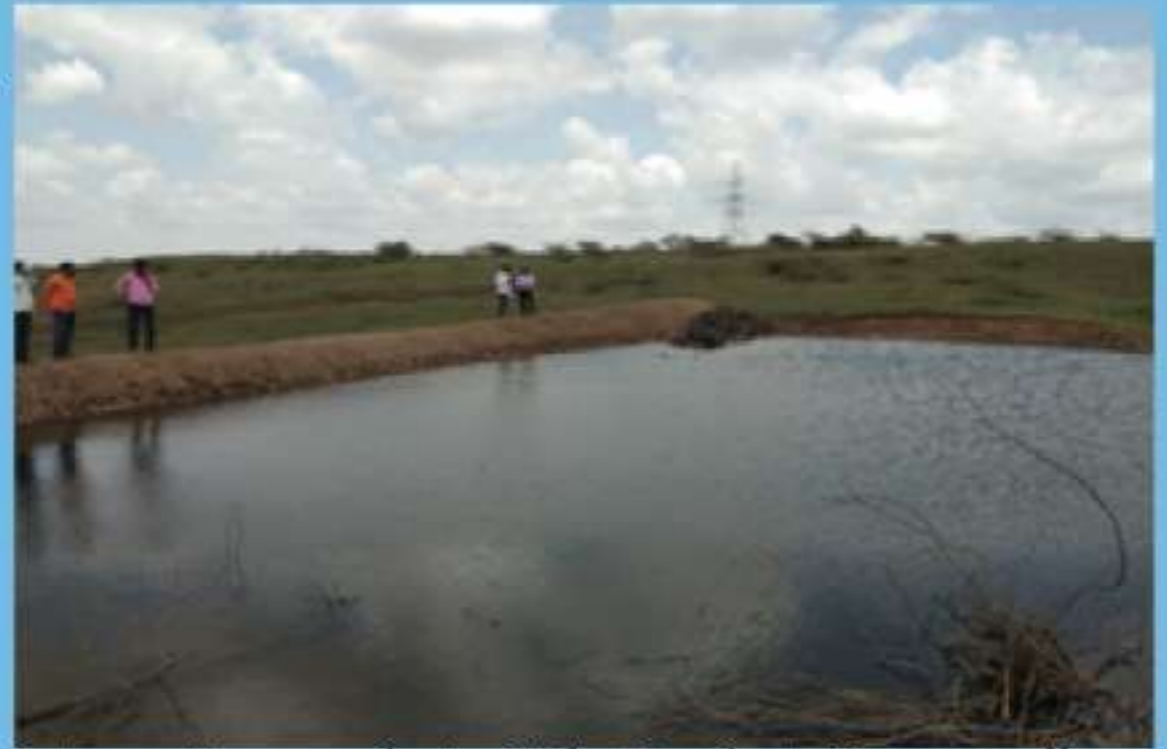
Interventions made in Nala Bund at Kannan village, Ethan block, Belgavi, Karnataka
