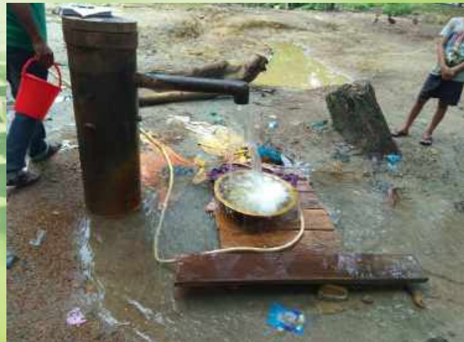
Autoflow well at Chandra Sadupara village, Jirania Block, West Tripura District.
