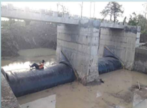
AjraPhata (Rubber Dam – Inflated Position)
