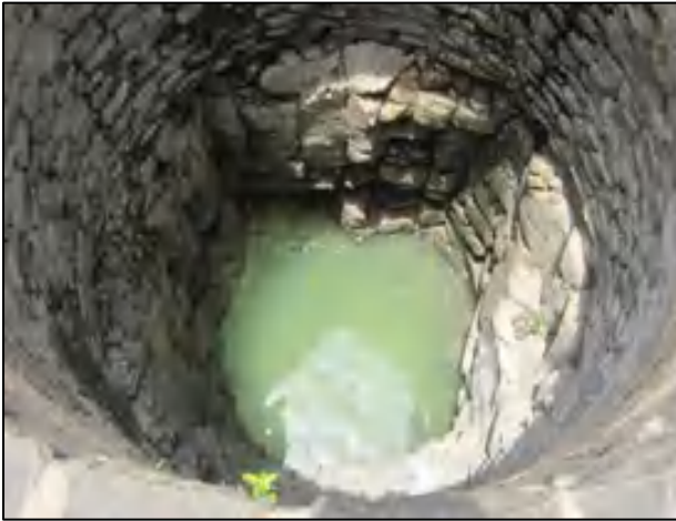
Fractured and jointed Massive Basalt (Aquifer-I) exposed in dug well section at Malegaon village, weathered basaltic zone has been lined by rock brick.
