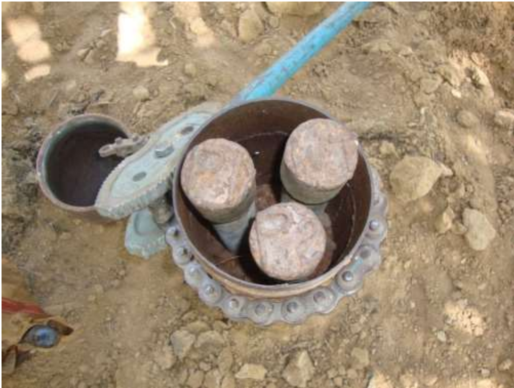
Existing piezometer nest constructed under VRB project in Byrapura village
