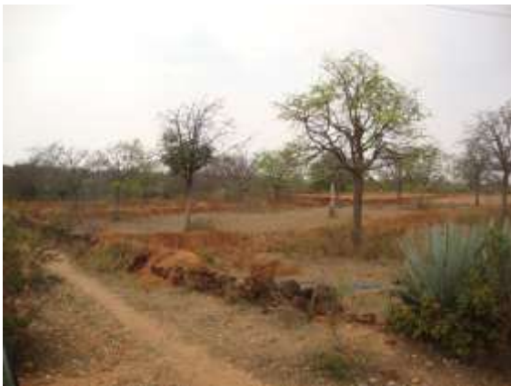
Construction of bunds at parcel on Bharanapura – Hosur road
