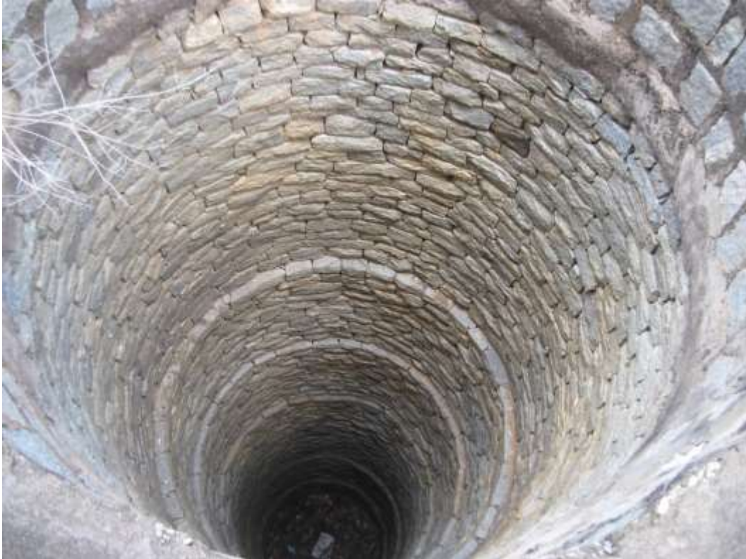
Dry dug well at Siddaramanagara village
