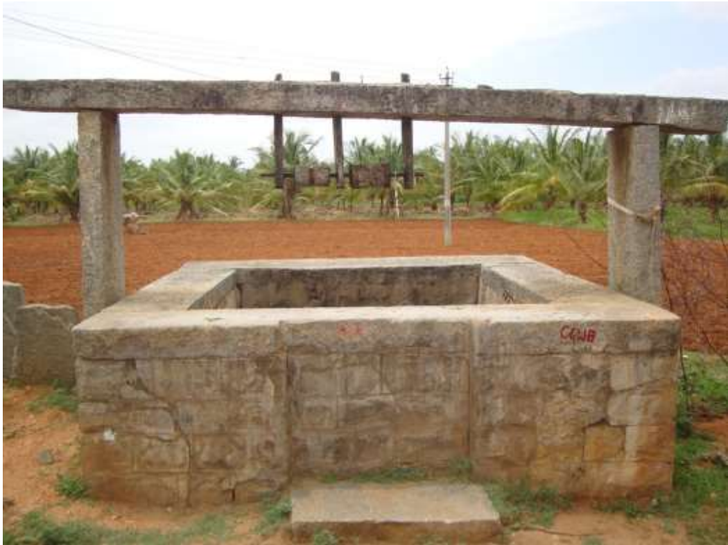
The typical dug well at B.Hosahalli village
