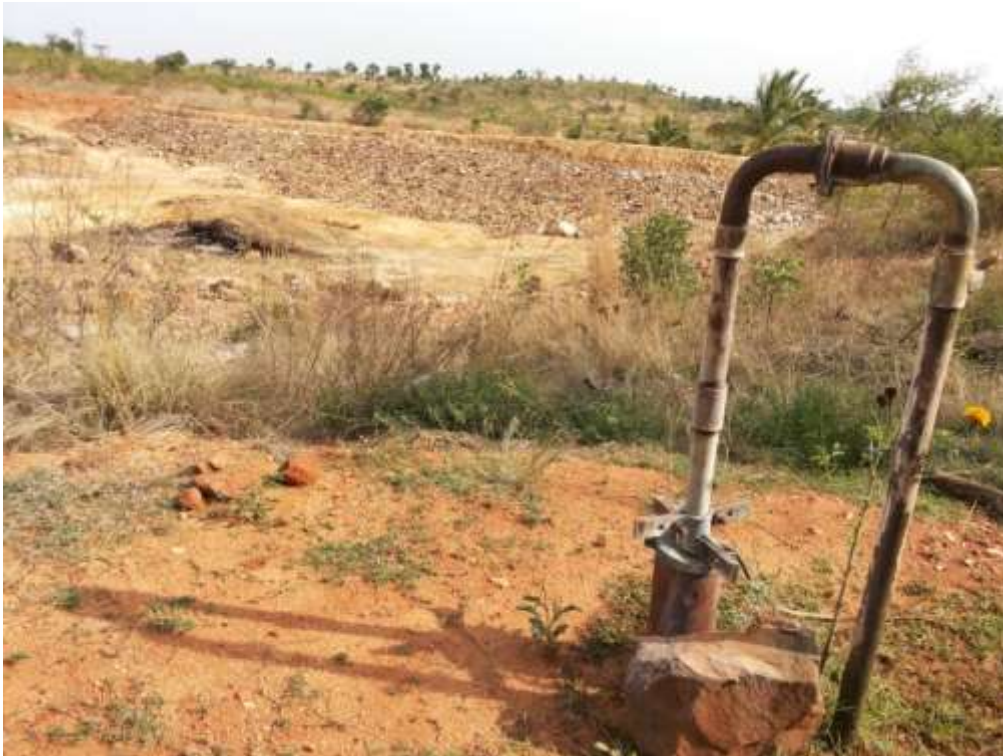
Check dam constructed across the third order stream near Kodalagara village
