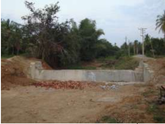
Check dam constructed accorss 3 rd order stream on Settikere – Dasihalli village
