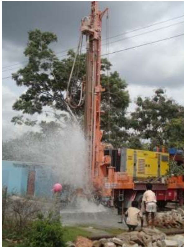
High drilling discharge encountered during drilling at Sasalu EW site
