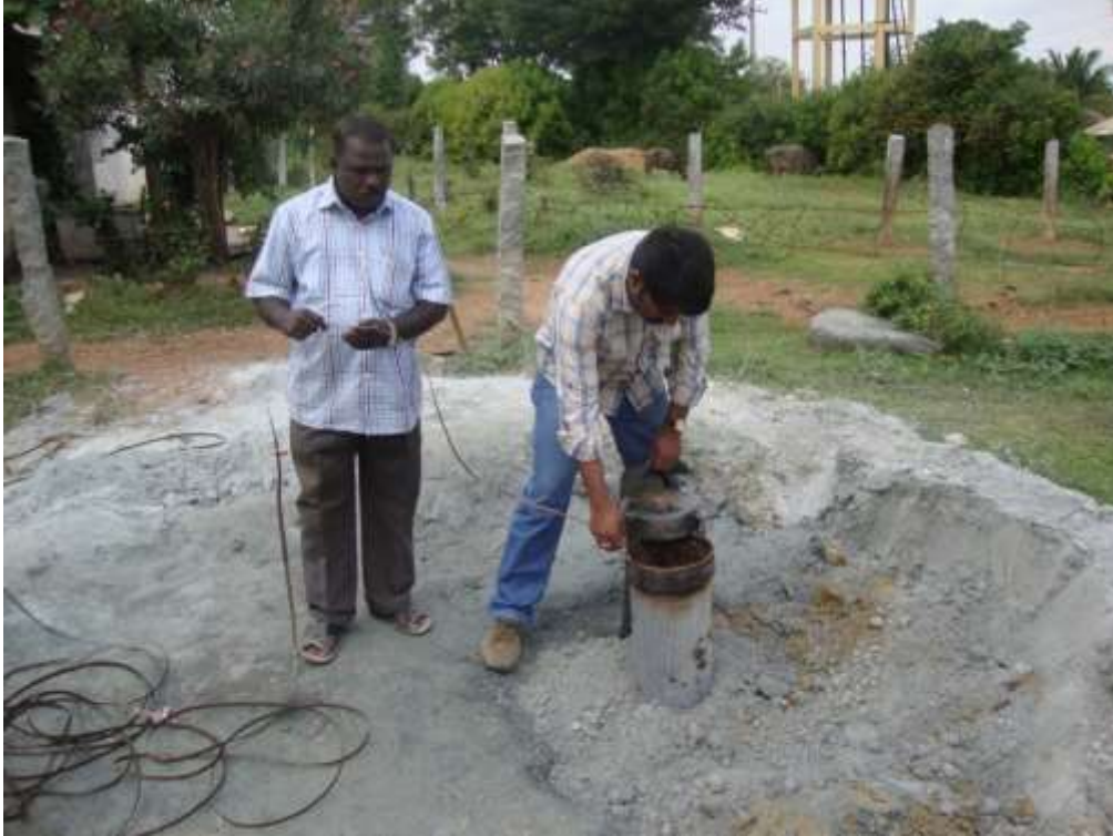
Monitoring of ground water level after completion of drilling at Huchanahatti EW site
