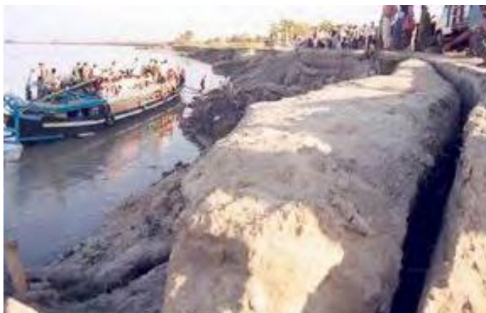
Fig.2 Erosion of Majuli Island by mighty Brahmaputra River
