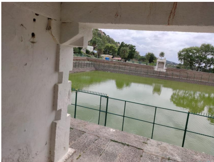
Photo 4: Large rectangular Temple well of Shivaganga temple tapping in phreatic aquifer Nelamangala Taluk.
