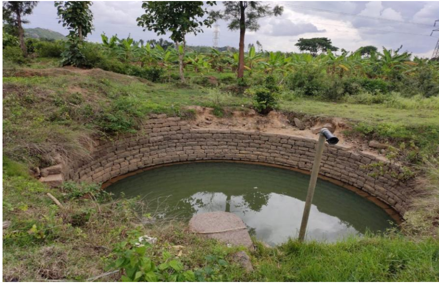
Photo 6 : A dug well with arrangement for recharge of surface run off at Sompura
