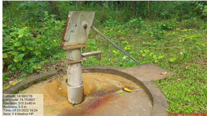
Photo 2.1: Hand pump where water is manually drawn in Madnur (14.98577, 74.7939)
