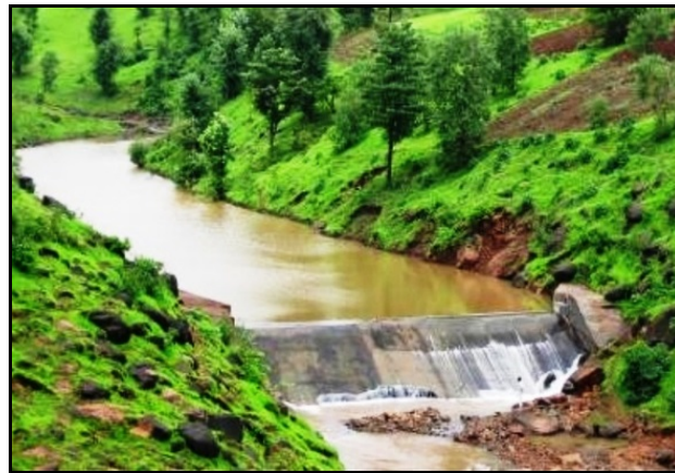
Figure 10.2 c : Illustrative Check Weir in Operation
