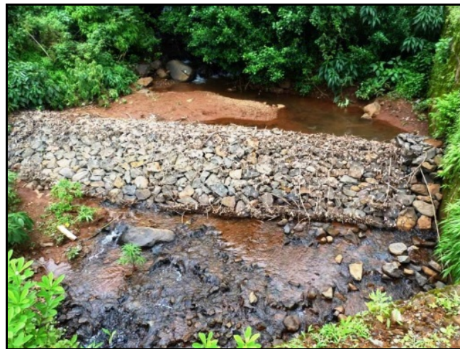
Figure 10.2 d : Illustrative Gabion Structure in Operation
