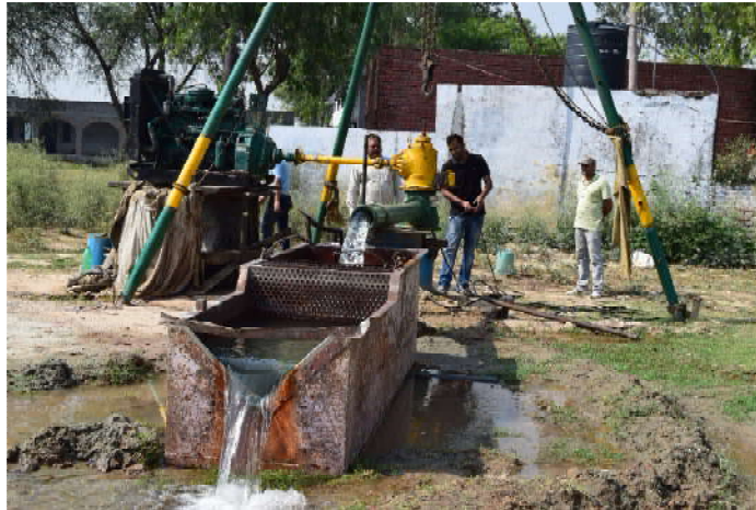
PUMPING TEST AT KHANPUR JATTAN (WELL FIELD)
