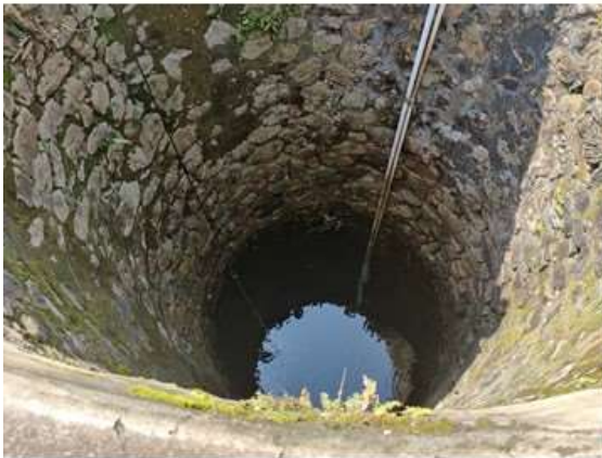
Stony walled dug well very common in the area
