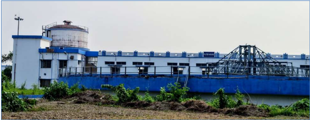
Water Treatment Plant of Public Health Engineering Directorate (PHED), Govt. of West Bengal at Dariapur, Kaliachak-III block. The plant is used for removal of Arsenic and also for rural water supply in Kaliachak-I, Kalaichak-II, Kalaichak-III and Manikchak blocks, Malda district
