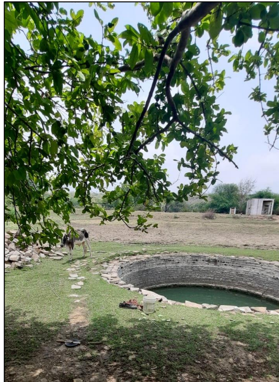
Figure 23: Dugwell at village Vikrampur showing shallow WL
