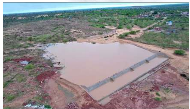
Check Dam, Village Sujannagar, block Balesar, district Jodhpur
