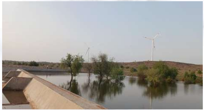
Check Dam, Bhalu Laxmangarh, Block Shekhala, district Jodhpur
