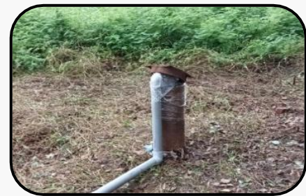
Use of unused borewells for groundwater recharge
