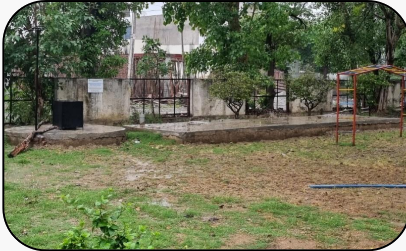
An Artificial Recharge System (Desilting Chamber, Filters and Recharge Borewell) in Faridabad
