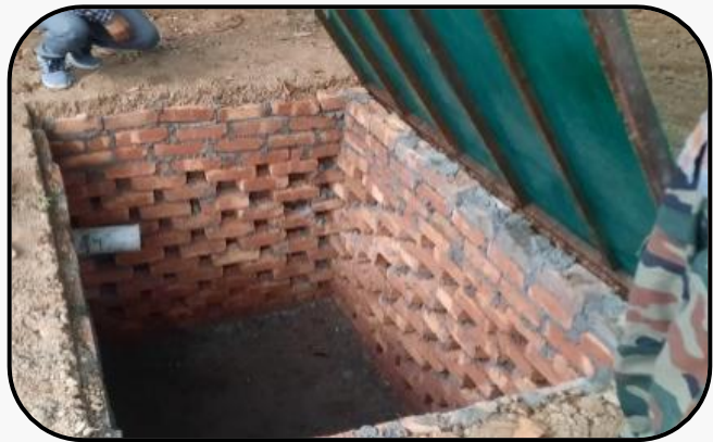
Sub-Surface Technique: Recharge Pit
