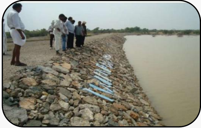
Surface Technique-Percolation Tank
