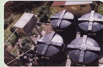
Harvesting of roof water in tanks
