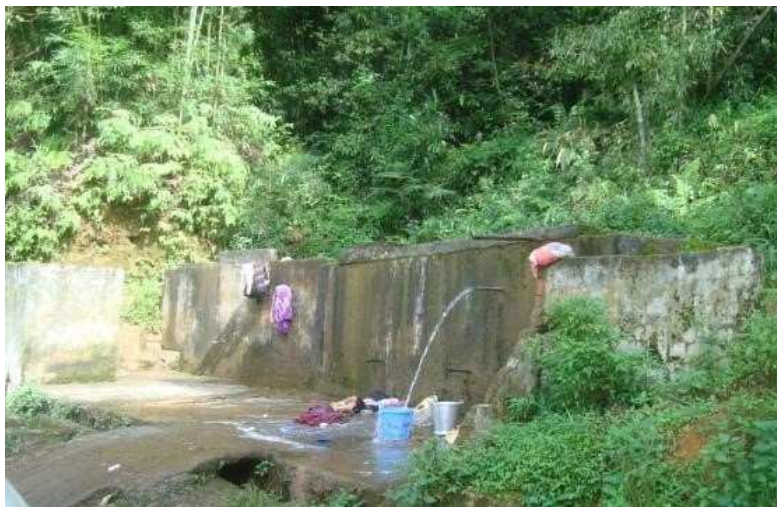
Fig10: Water from Contact spring being collected by constructing spring tap chamber at Ri-Bhoi District. CGWB
