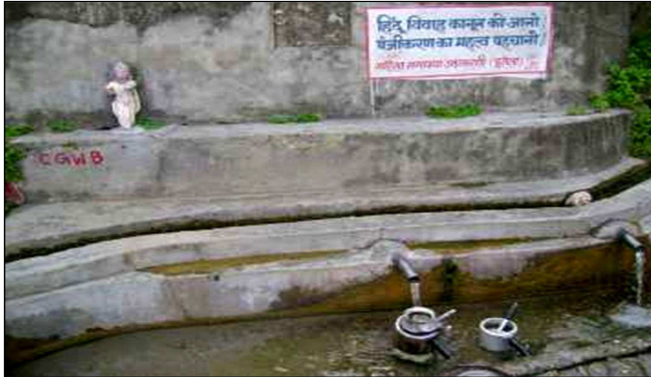
Fig.18: Spring source tapped through channels for water supply at Khalari village, Purola block, Uttarkashi district (Photo CGWB)
