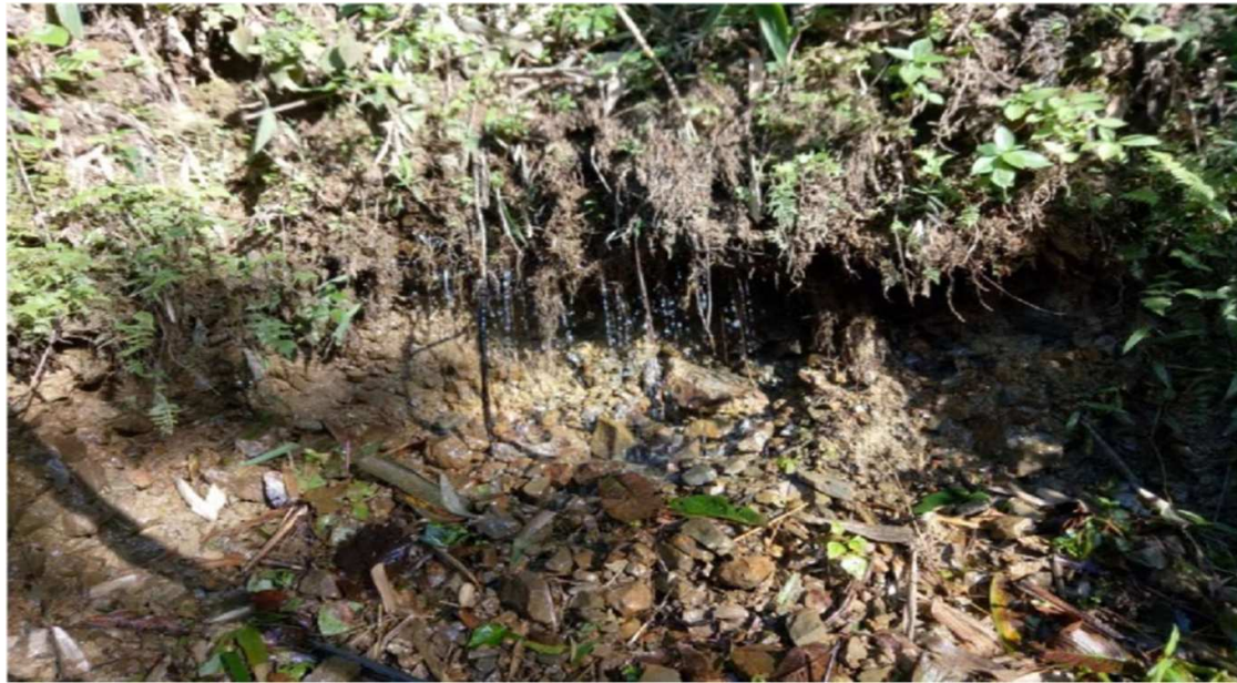
Fig3. Ground water seepage in Kohima District, Nagaland (CGWB)
