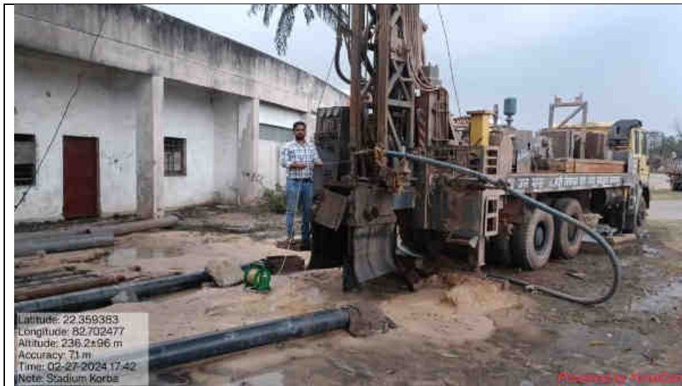
1. Hydrogeological Test for Piezometer Construction in Indira Stadium, Korba
