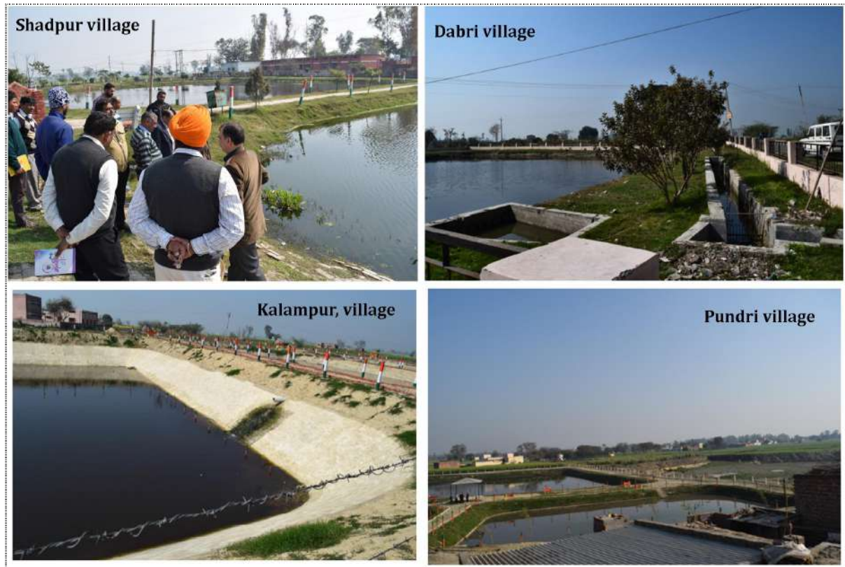
Figure-33: A view of village tanks of five pond / three pond system of water treatment under natural process.
