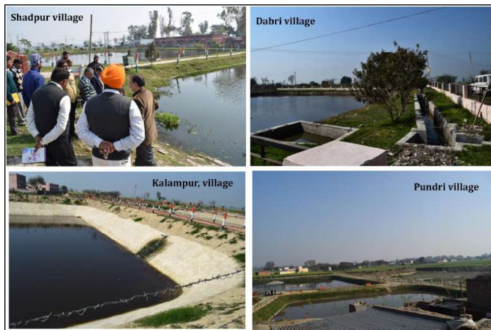
A view of village tanks of five pond / three pond system
