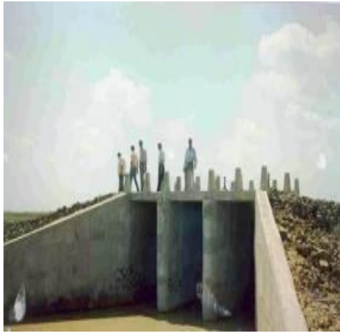
Fig-4.4: Sluice gate under construction at the creek entrance
