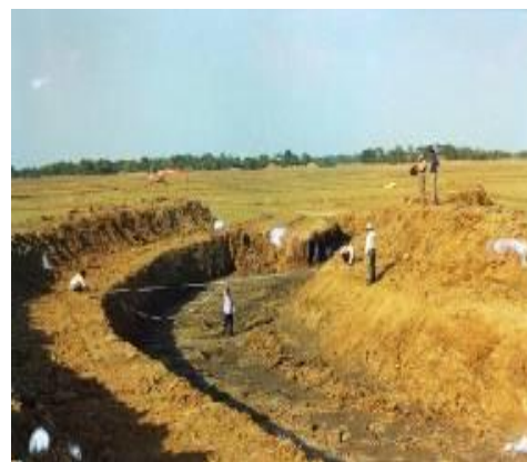
Fig -4.3: Renovation (deepening & widening) of Creeks underway
