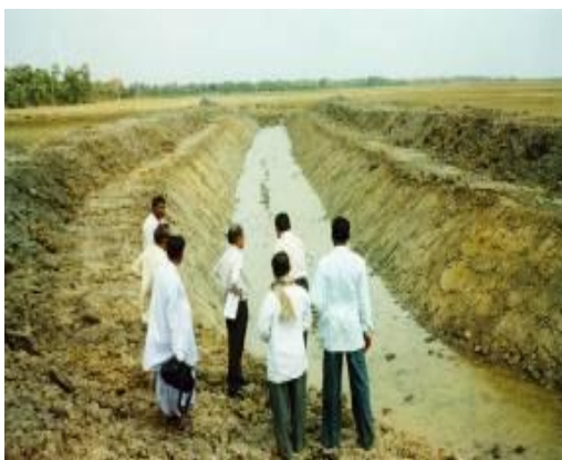
Fig -4.3: Renovation (deepening & widening) of Creeks underway
