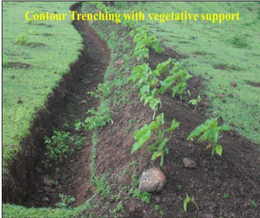
Fig.8.2.1a Section of a Contour Trench
