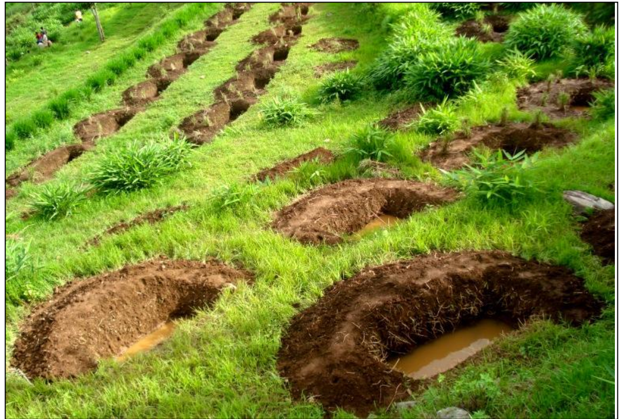
Fig.8.2.1b Staggered Trenches
