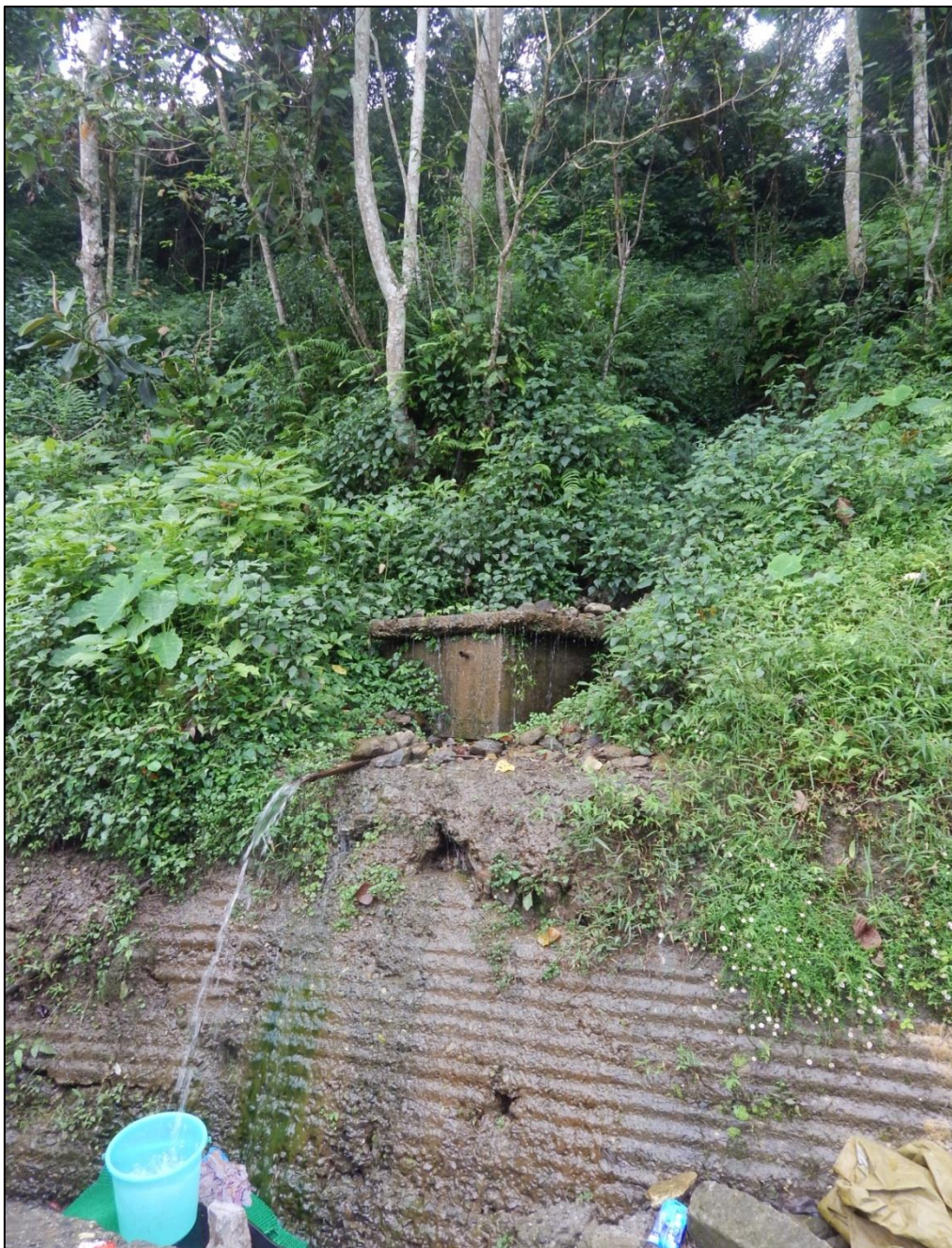
Fig.8.2.4a Spring Box in Namthang block, South Sikkim district
