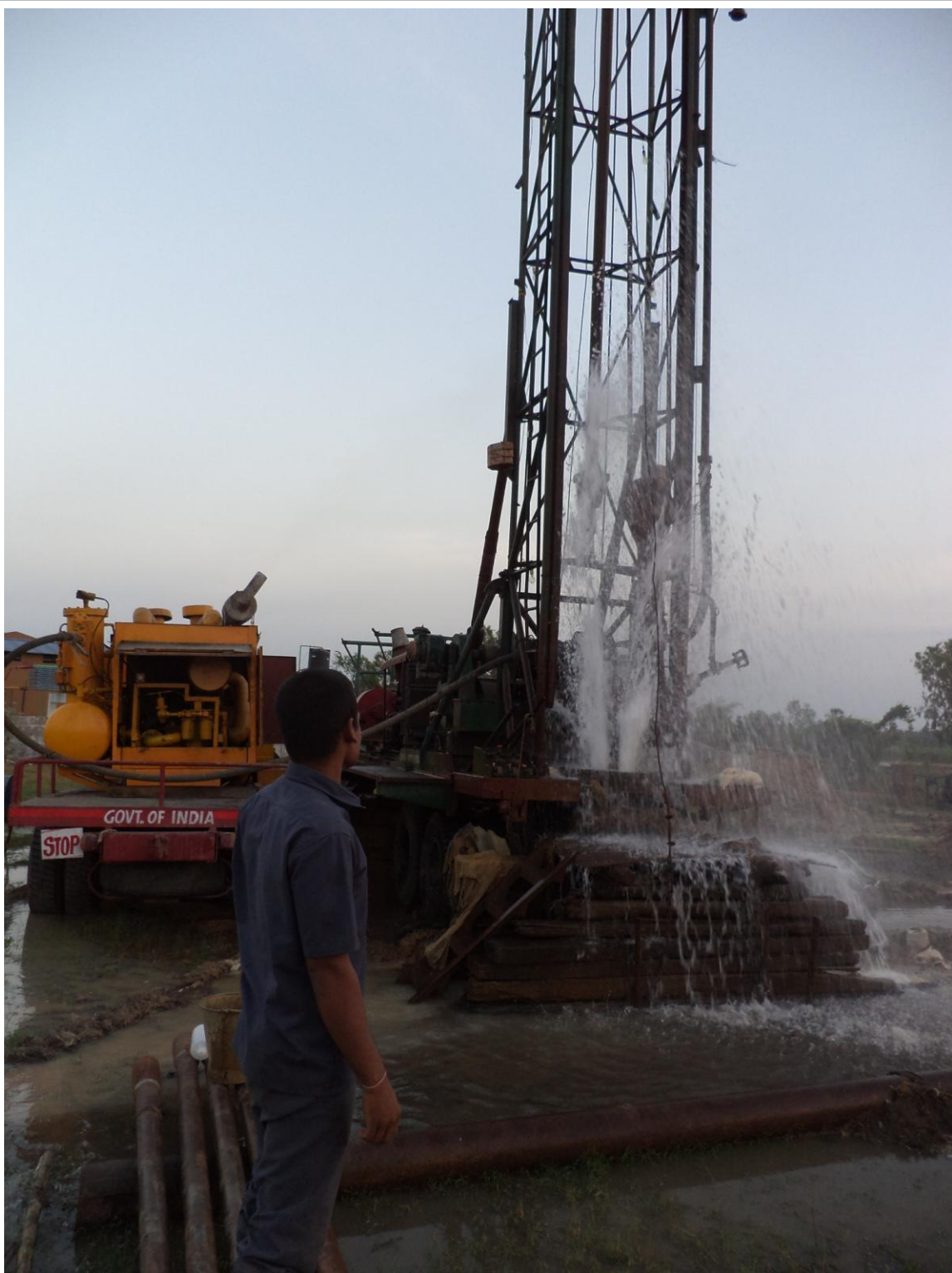
Fig 2.1 Well development at Ayekuppam site, Cuddalore dist (Exploratory Drilling at Pilot Project site – lower velar water shed)
