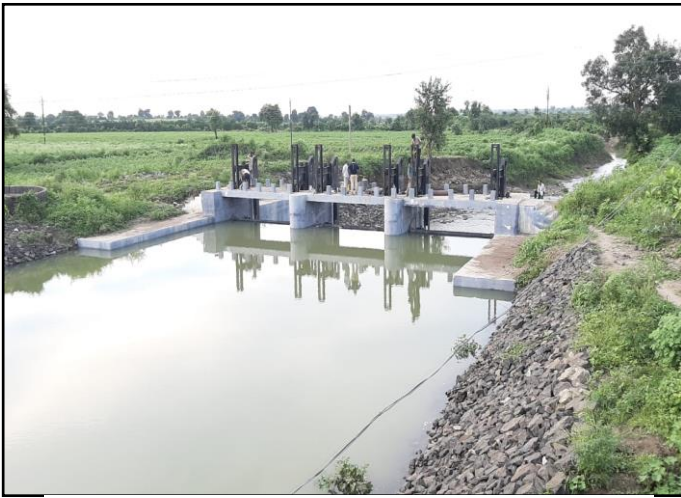
Sarwadi (Gates in closed position)
