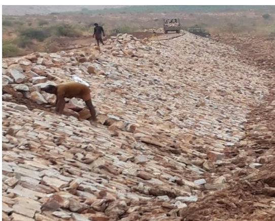
Fig.10.4 Percolation pond under construction
