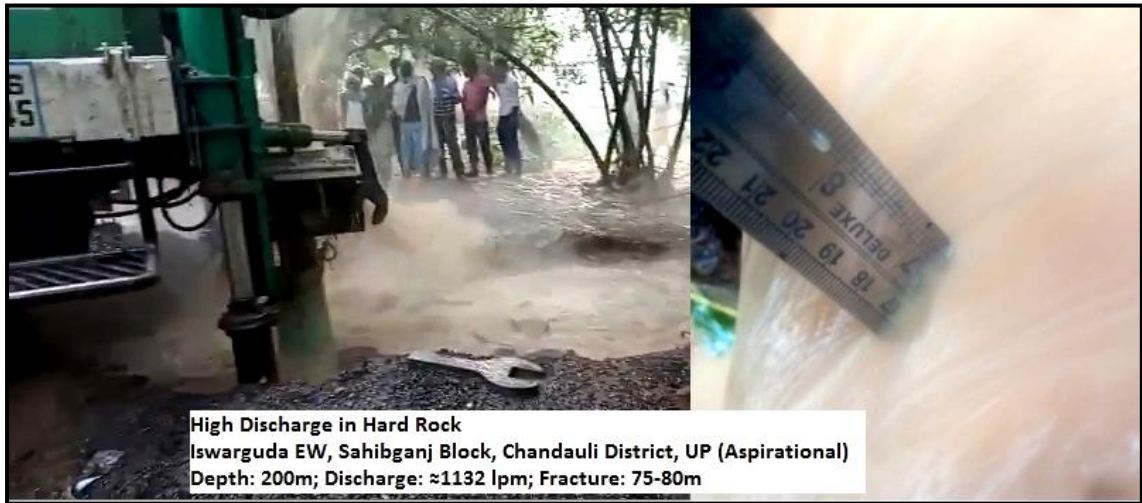
Fig.3.3. High discharge of ≈1132 lpm has been obtained from the Exploratory Well drilled (Depth: 125m; Fractures: 75-80m) in Hard Rock at Iswarguda, Sahibganj Block, Chandauli district (Aspirational), UP
