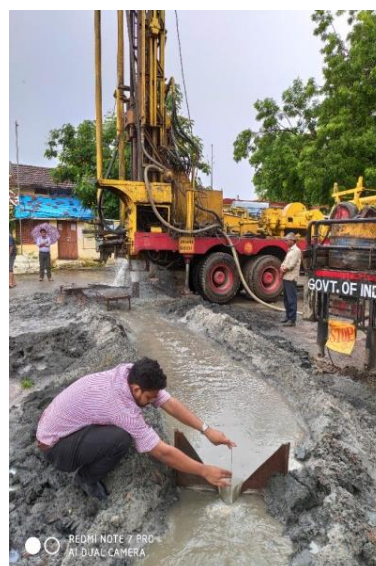
Fig. 3.2 EW drilled to a depth of 160 mbgl at Dahegaon village in Samudrapurtaluka of Wardha district, Maharashtra yielded a discharge of 465.6 lpm
