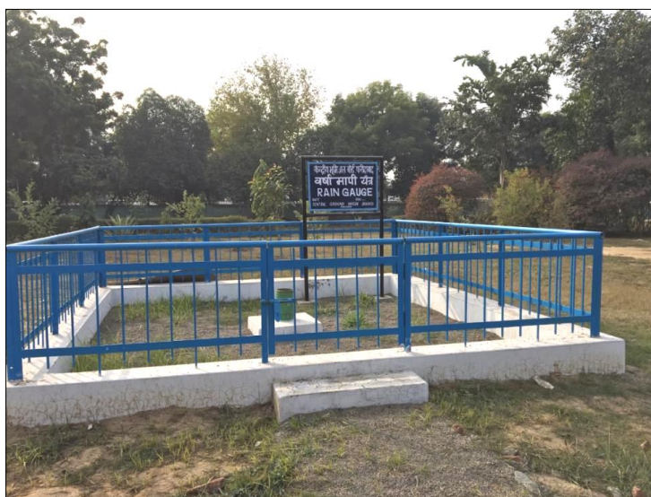
Fig. 6.1 Raingauge structure in Bhujal Bhawan, Faridabad campus
