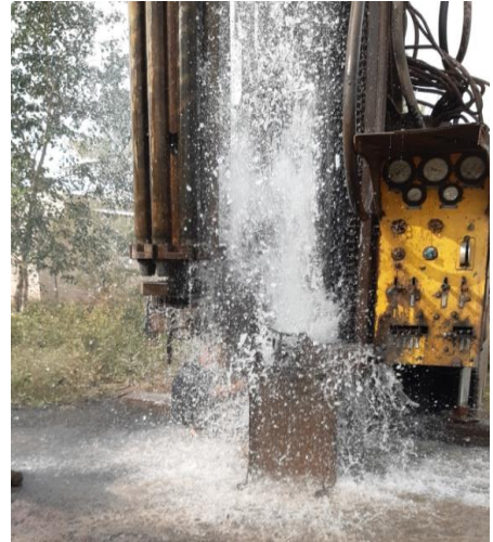
Fig.3.6: Exploratory well drilled down to a depth of 160 m bgl at Samarthgaonin Satarataluka of Satara district, Maharashtra state has yielded a discharge of 12.18 lps in Deccan basalts
