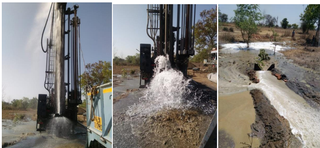
Fig.3.4: High Yielding Well at Borda, Ramtek taluka, Nagpur district, Maharashtra State drilled down to a depth of 160.00 m bgl with discharge of 480 lpm.
