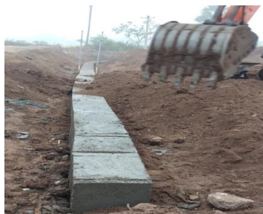
Fig.10.5 Sub-surface barrier under construction
