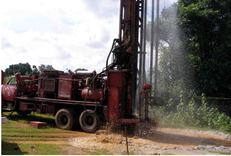
High yielding (25.00 lps) bore well drilled at village & block Kalebira, Simdega district
