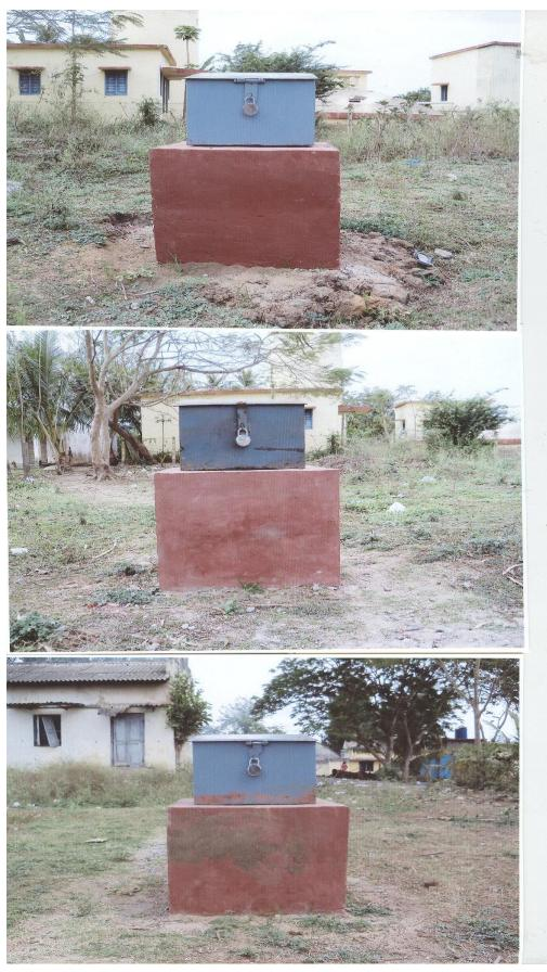
Protection Box (Plate thickness GI sheet -. Annexure-Q 3.00 mm) 65 CM 65 CM 53 CM 45 CM 55 cm 55 CM 25 mm ¢ holes **Bottom Side** 10CM 55CM 35CM X 5 CM 10CM 65 CM 5 mm Heavy duty Hinges Heavy duty pad lock SIDE VIEW
