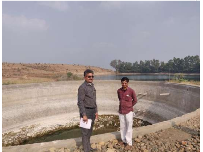
A view of large dia dugwell (26.5 mtrs.) being used for water supply in the village.
