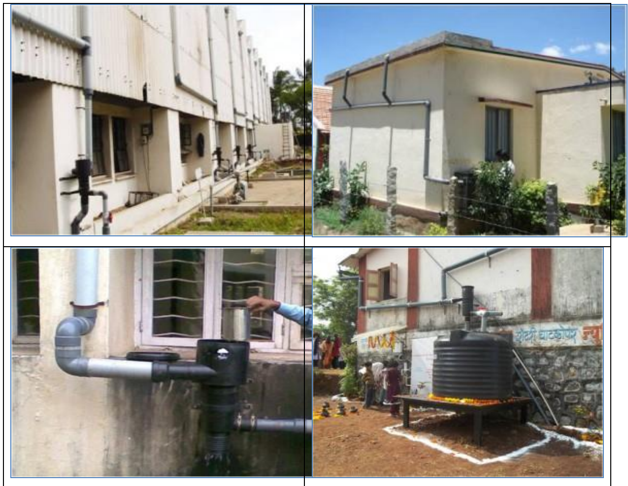
Fig 6.5 Storage Tank (for direct use)
