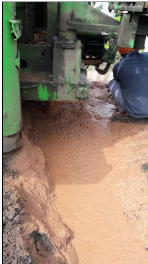
Red bole encountered (93 to 102 m bgl) at EW at Pangarkhed, Malegaon Taluka, Washim district
