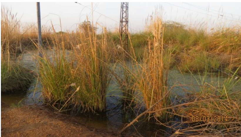
Plate 2. Water logging situation along IGNP Canal, Ramgarh area, Jaisalmer district, Rajasthan
